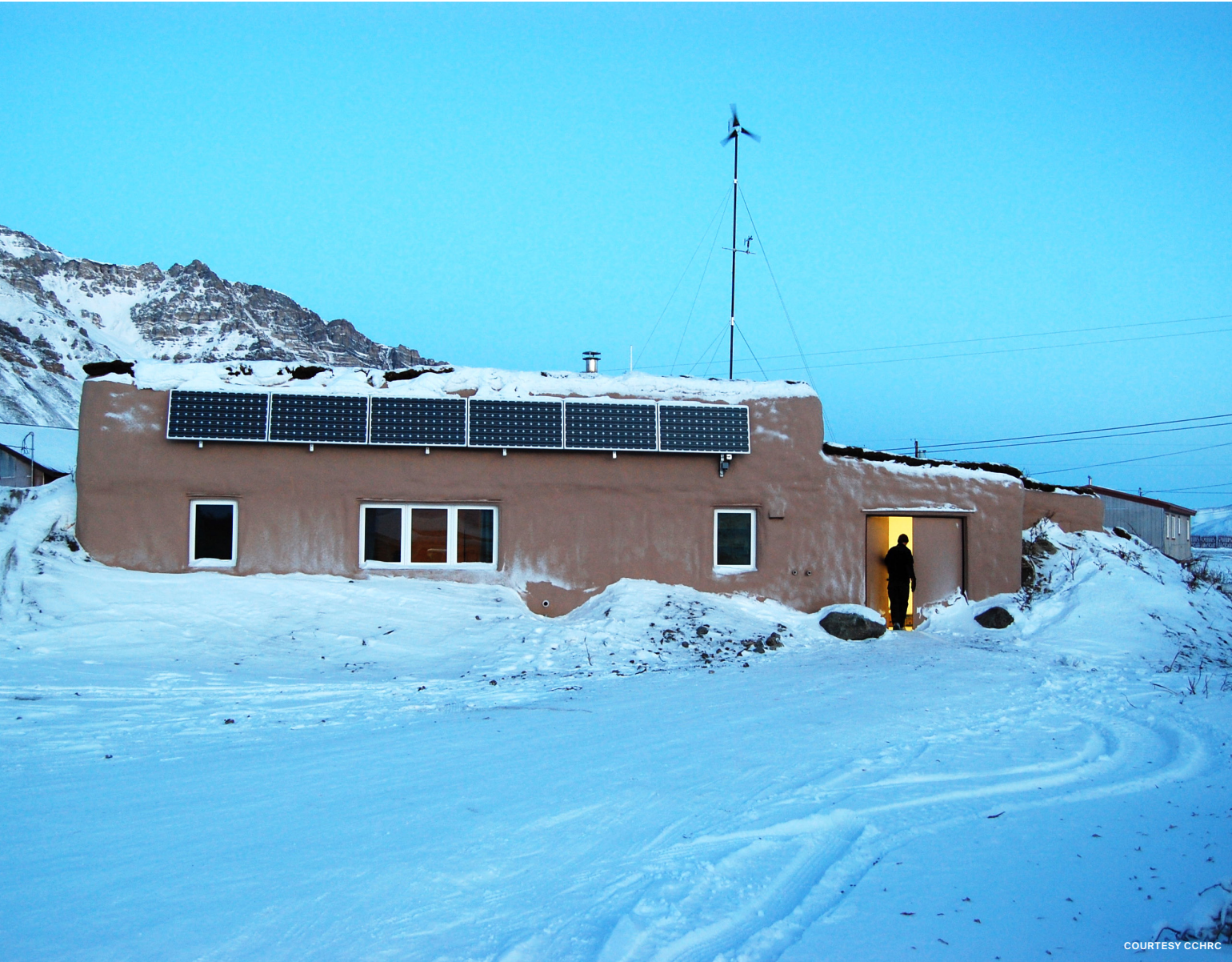
A house in Anaktuvuk Pass, Alaska, where unexpanded spray-foam was flown in and used to create an “inside-out” wall assembly system with metal studs covered in the foam insulation. It was designed with material transport costs as a driving force.
