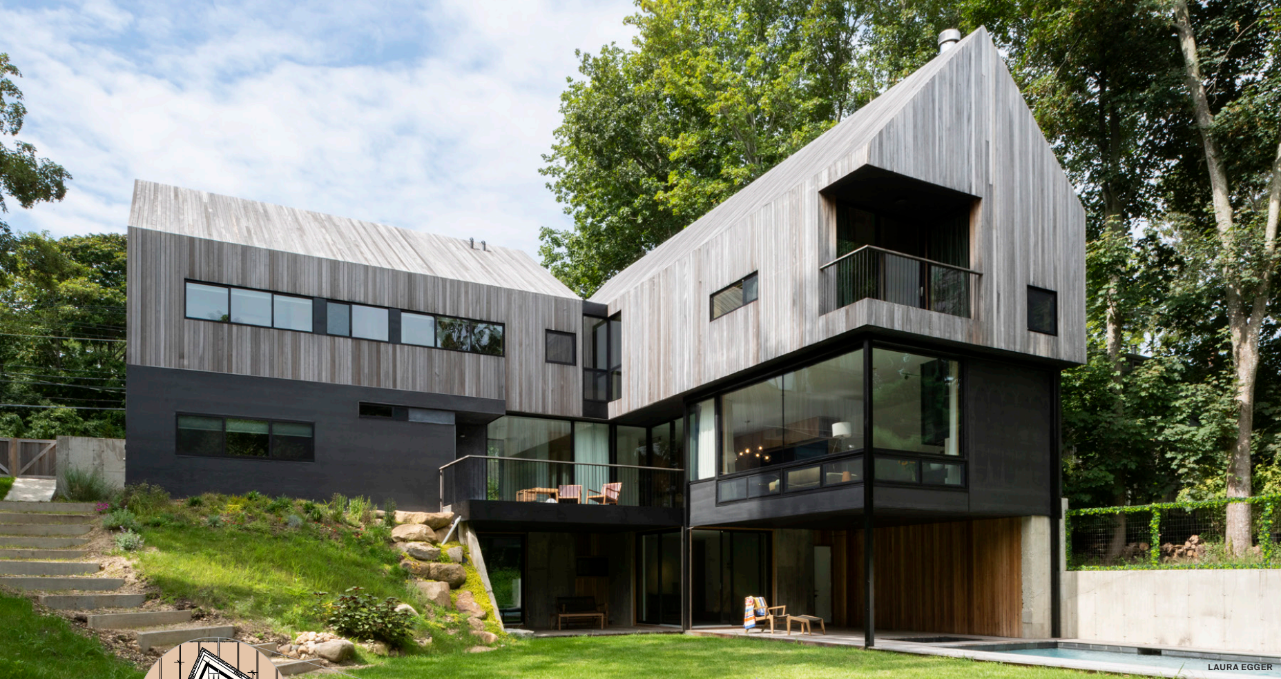
Above: The exterior is clad in mahogany, birch, and EPDM rubber, each material covering a separate floor. Left: The building’s multiple cladding materials required a range of section and corner details.
