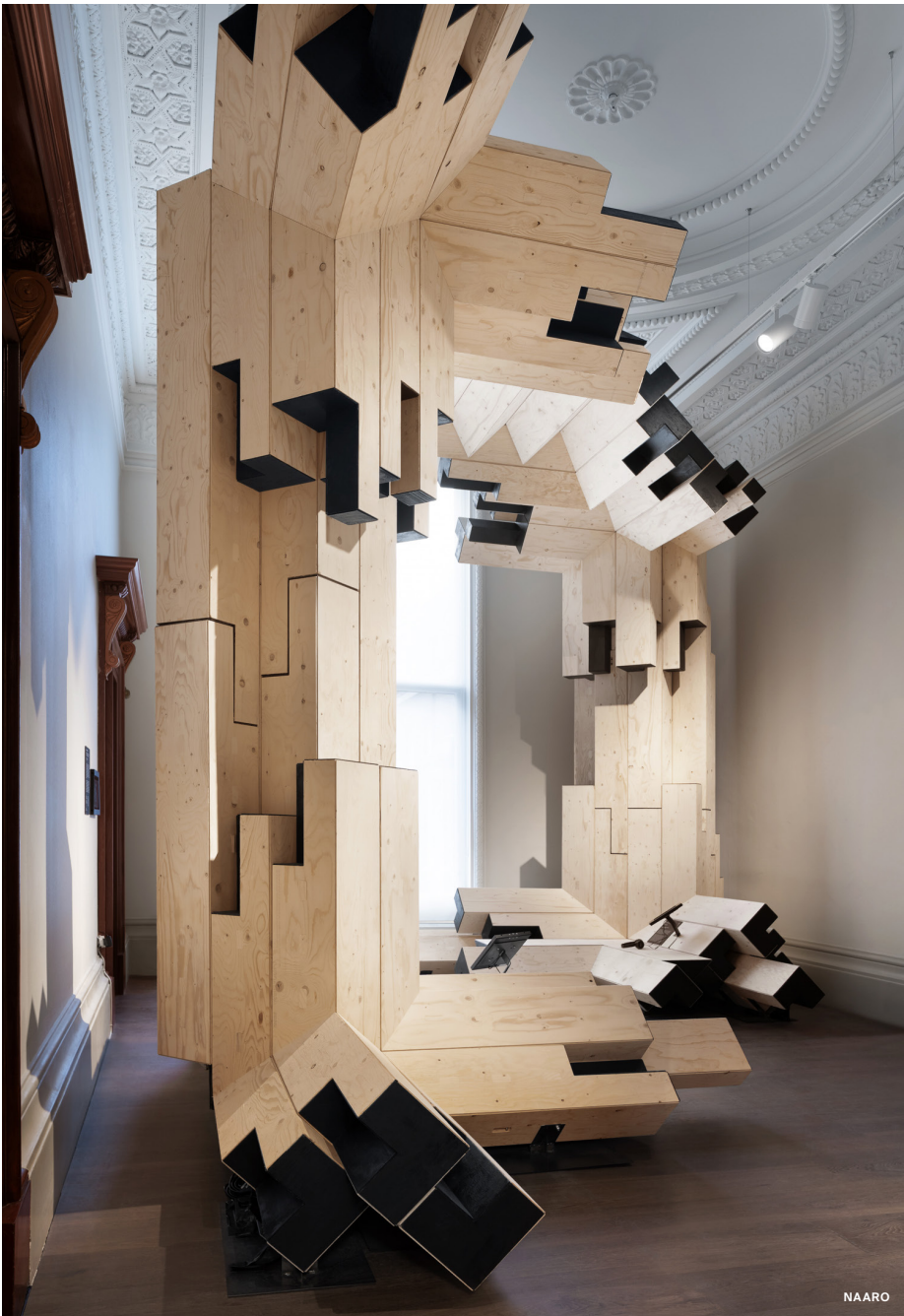
Retsin's team used augmented reality to assemble a pavilion at London's Royal Academy.
