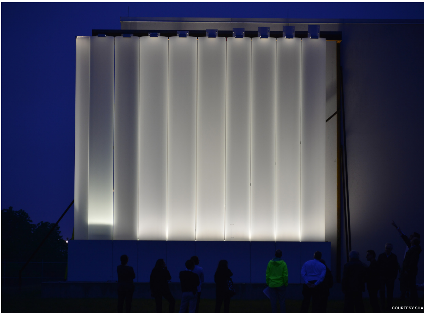
The design concept for the glass rain screen was to establish translucency with depth. The result is a lamp-like effect of trapped light.
