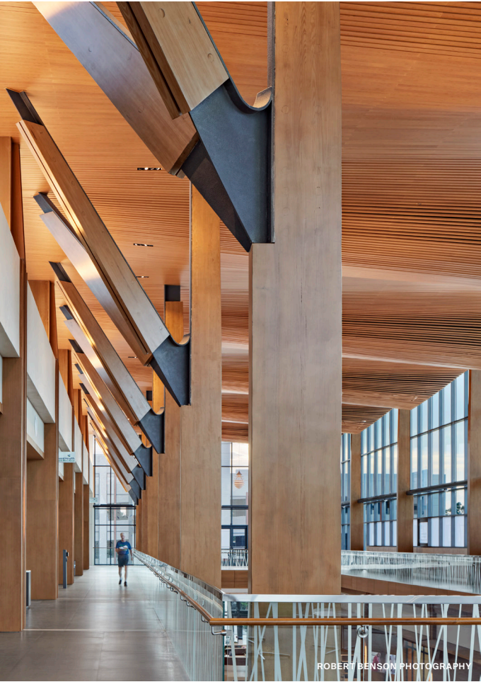
Below: Gardens and natural materials support the center's wellness and mental health missions. Left: Glulam columns from Bell Structural Solutions hold up a soaring roof.
