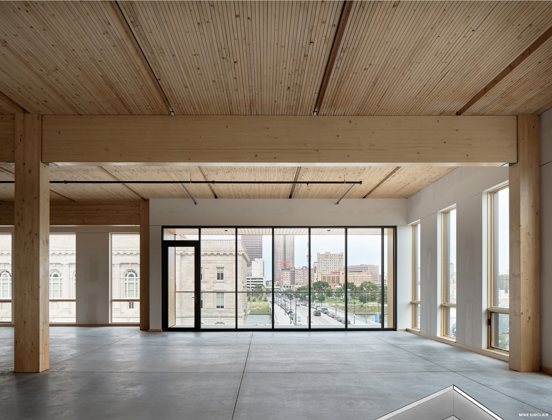
The layers in the laminated timber create a striated ceiling pattern.
