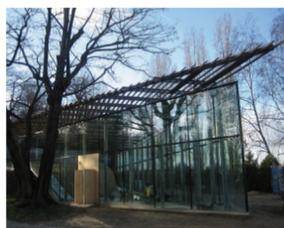
The chapel is enclosed within a lightweight glass structure (left) made of a DuPont SentryGlass Plus structural interlayer laminated with SGG Stadip safety glass from Saint-Gobain Glass. The interior of the chapel and the overall triangular shape (left) retain the same raw but intimate sensibility of the original tent structure. The interior chapel (above) is an upturned wooden shell clad in pine strips individually steam-curved on site.
