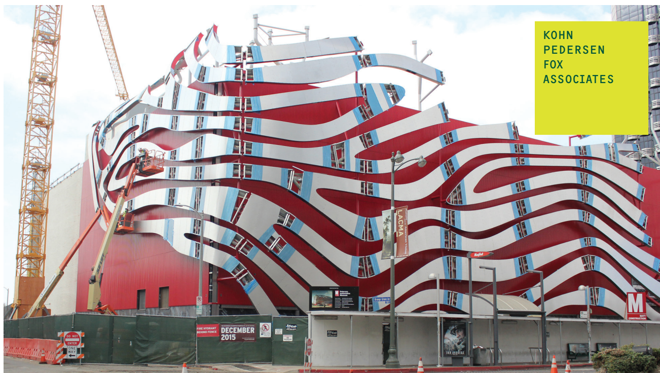
All wrapped up and tied with a bow: Stainless steel ribbons designed by KPF and fabricated by Zahner were craned into place in 25-foot sections. The design pays homage to sports cars and chrome detailing.
