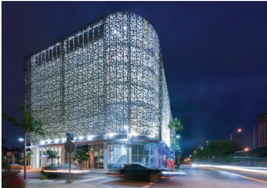
3D PERFORATED METAL ZAHNER One of Zahner’s classic facade manufacturing techniques has now become streamlined thanks to its automated method for creating perforated louvered screen wall facade systems. Now it is easy to create picotage effects for architectural metal that allow airflow without harsh sunlight. azahner.com
