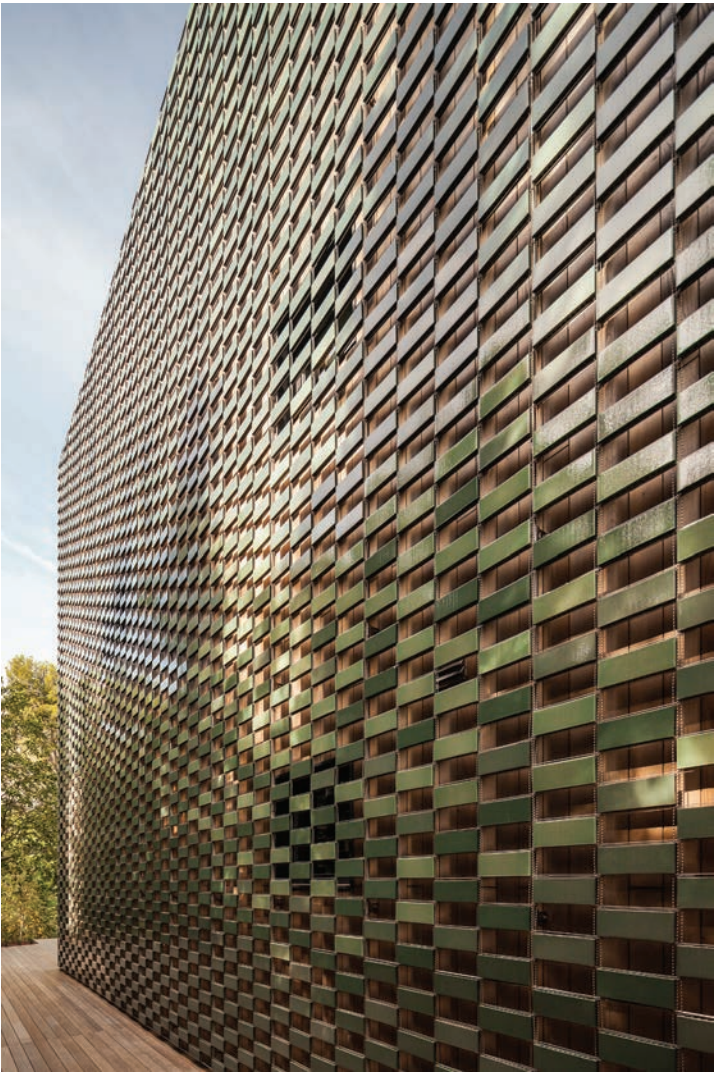
FABRIK SHILDAN FOR FLEXBRICK Fabrik is very much like a textile for exterior architecture. It consists of a steel framework into which materials are woven (including terra-cotta, glass, wood, etc.) to create endless patterns in a flexible architectural mesh. In addition to facades, Fabrik can be used for pavement, roofing, shade screens, and more. flexbrick.net
