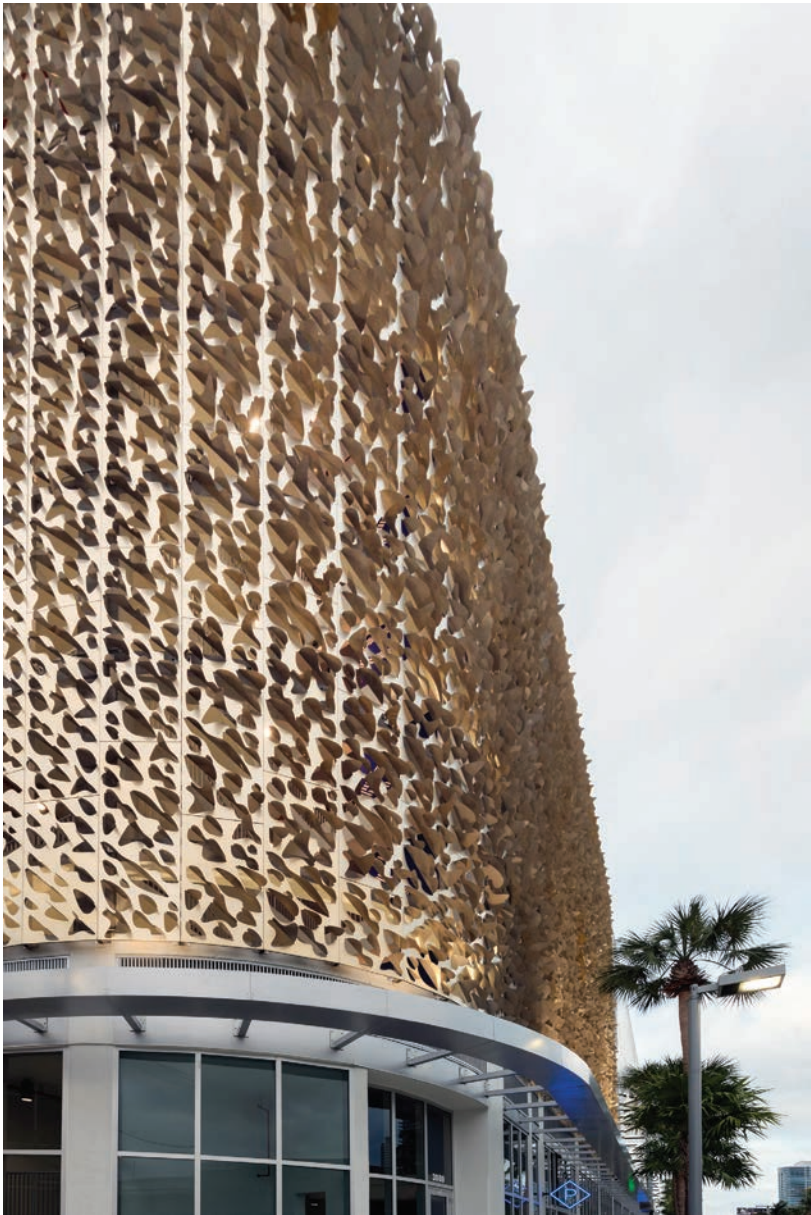
3D PERFORATED METAL ZAHNER One of Zahner’s classic facade manufacturing techniques has now become streamlined thanks to its automated method for creating perforated louvered screen wall facade systems. Now it is easy to create picotage effects for architectural metal that allow airflow without harsh sunlight. azahner.com
