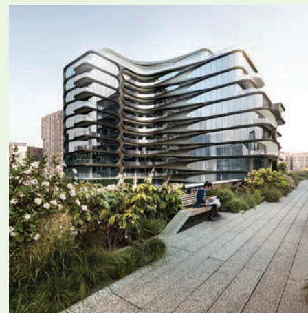
Courtesy Zaha Hadid Architects
