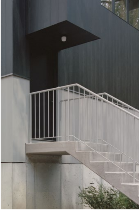
ABOVE AND RIGHT The Ardmore House in Chicago, with gray and black Accoya wood cladding
