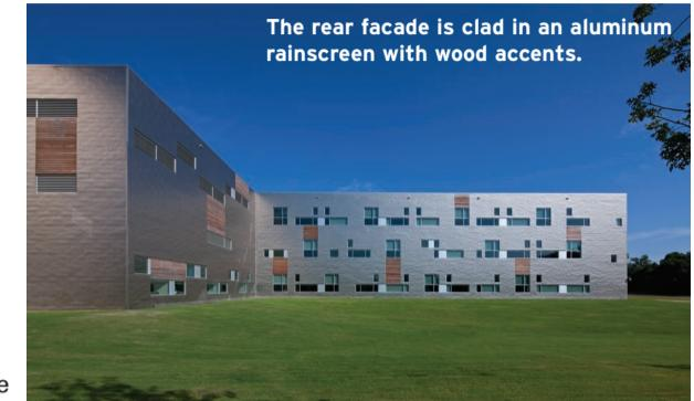
The rear facade is clad in an aluminum rainscreen with wood accents.
