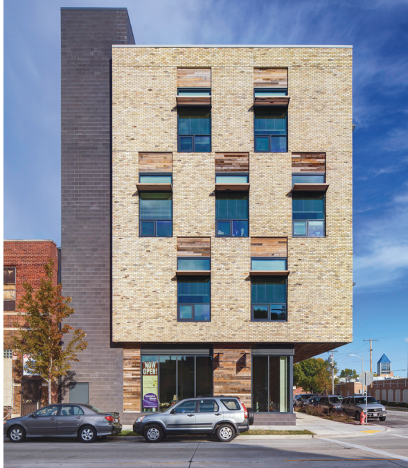
The building uses reclaimed brick (left) and pickle barrel wood (above) and boasts a rooftop farm (below).
