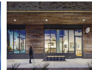
The building uses reclaimed brick (left) and pickle barrel wood (above) and boasts a rooftop farm (below).
