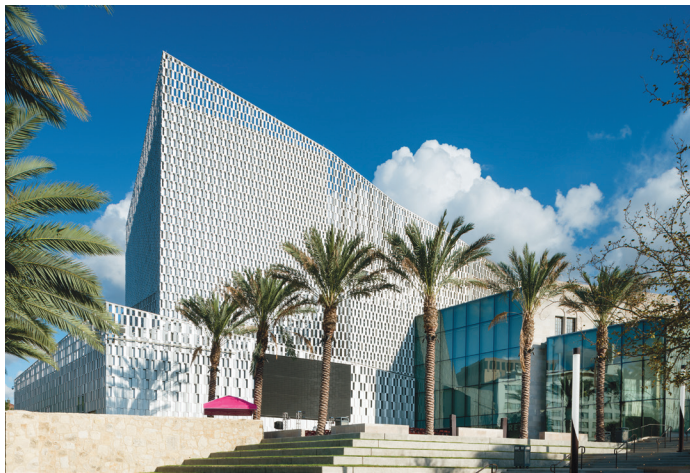
The architects preserved the historic Spanish Mission Facade of the Municipal Auditorium, while cladding the new building elements in perforated metal panels with integrated LED lighting.
