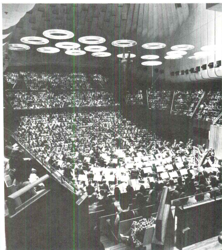
Plastic doughnuts float above the audience and improve the sound
