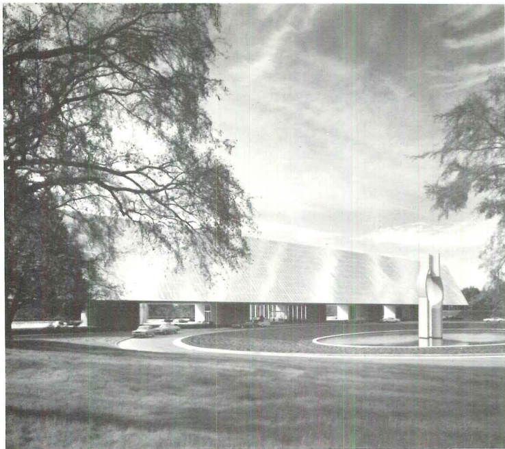
Tilted mirror glass facade facing north
