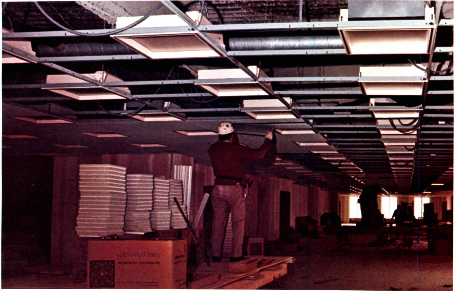
Approximately 2½ million sq. ft. of ceilings utilizing Roper Eastern's Tab-Lock 281 acoustical grid suspension system. Standard Oil Bldg., Chicago. Contractor: McNulty Bros. Co.
