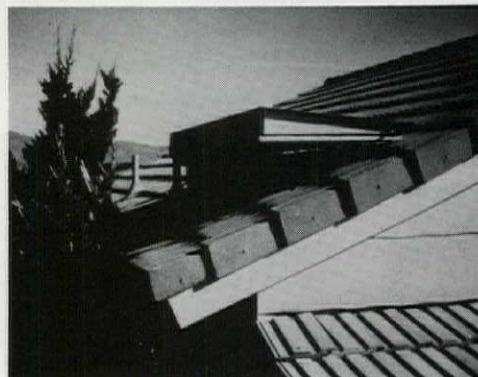
Combined solar still and hot water heater
