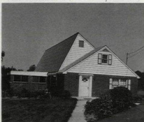
Thomason's solar heated and cooled home
