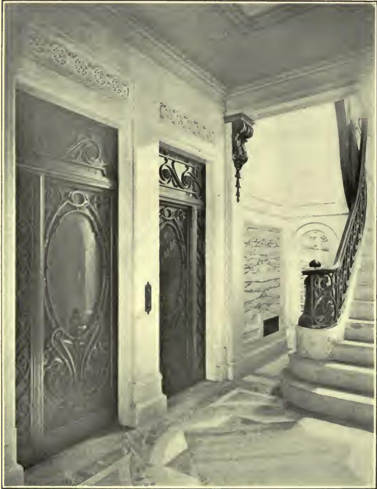
BRONZE-FINISHED IRON STAIR RAILING AND ELEVATOR ENCLOSURES.
