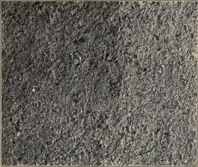
FIG. 8. SAND BLAST TREATMENT OF CONCRETE SURFACE.
