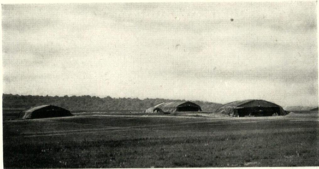
Plate F. Bessoneau hangars shown in plate B. In the right hand shelter may be seen the tail of a plane. The camouflage covering is stretched down over the side supports so as to eliminate tell-tale shadows. See plate G for detail of Bessoneau hangar.
