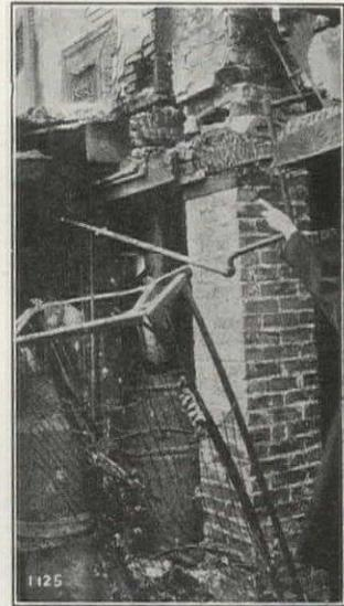
Chimney without Flue Lining. See where the brick dropped out and the fire started.
