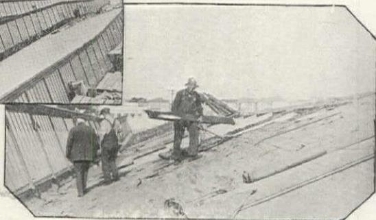
Roof boards of Redwood prevent condensation of moisture, as well as resisting decay-producing fungi
