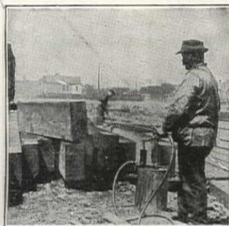
Spraying: Applying Carbosota to ends, mortises and tenons (points of contact) of caps and stringers for trestle.
