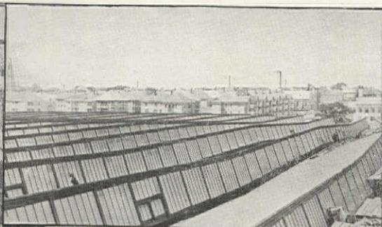
Saw-tooth roof Whitman Weaving Mill, New Bedford. Rotted boards replaced with long-lived Redwood
