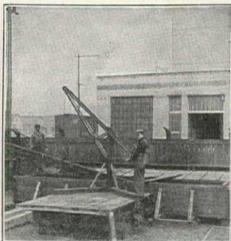
The Open-Tank Process: Simple wooden tank (lined with sheet iron), equipped with steam coils and small derrick.
