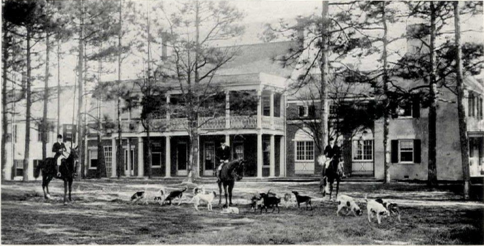
THE JAMES BOYD HOUSE, SOUTHERN PINES, NORTH CAROLINA Aymar Embury II, Architect
