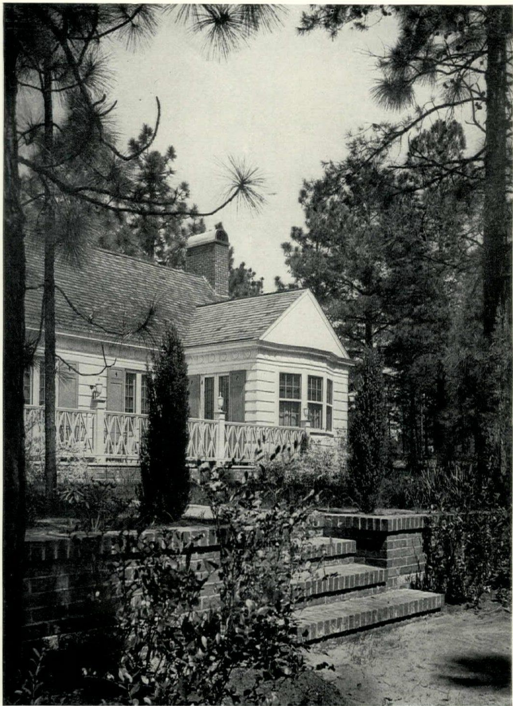
Detail of Front Elevation THE DR. E. E. CADY HOUSE, SOUTHERN PINES, NORTH CAROLINA Aymar Embury II, Architect
