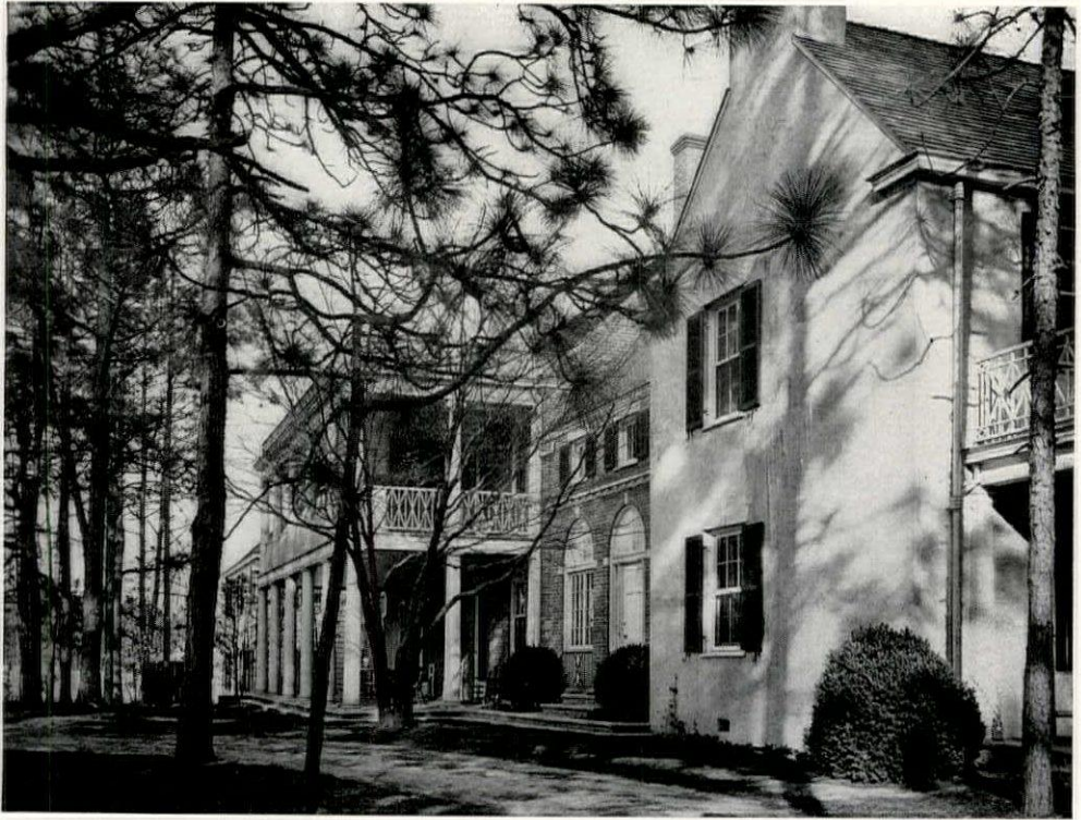
THE JAMES BOYD HOUSE, SOUTHERN PINES, NORTH CAROLINA Aymar Embury II, Architect
