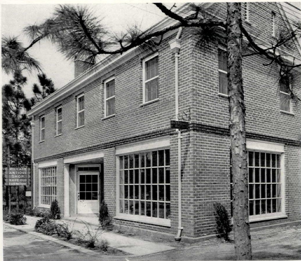
"CLIFTON CHAMBERS," PINEHURST, NORTH CAROLINA Aymar Embury II, Architect
