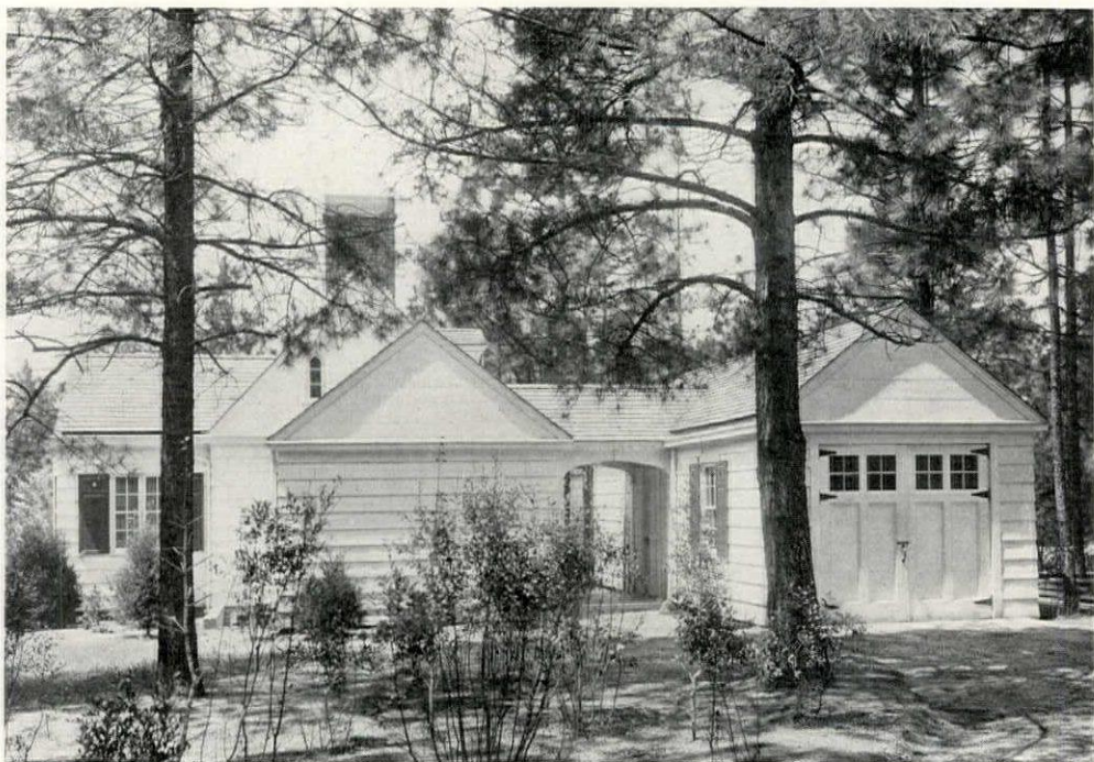
SIDE ELEVATION AND GARAGE—THE DR. E. E. CADY HOUSE, SOUTHERN PINES, N. C. Aymar Embury II, Architect
