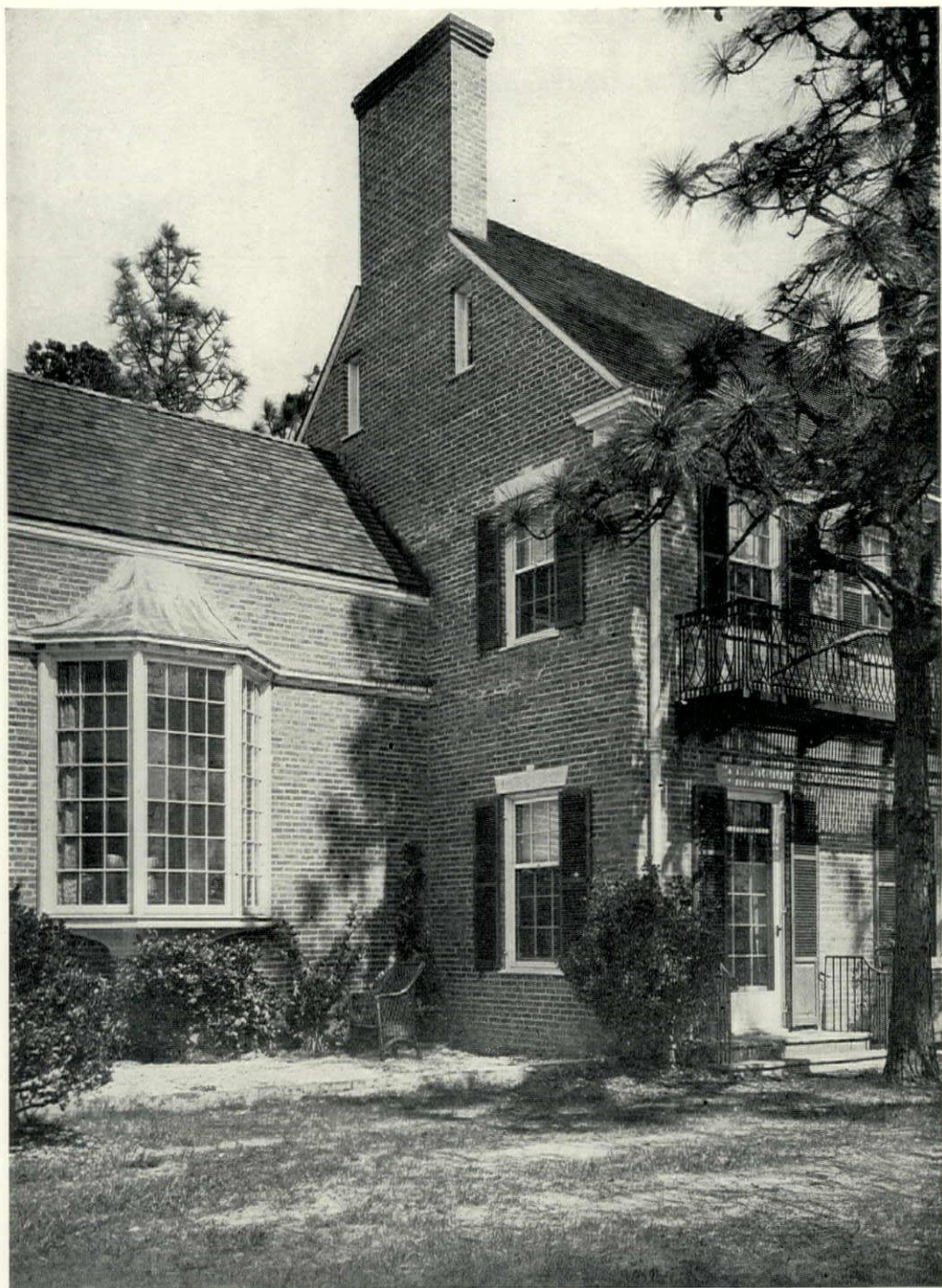
Detail of Bay Window and Rear Elevation THE JAMES BOYD HOUSE, SOUTHERN PINES, NORTH CAROLINA Aymar Embury II, Architect
