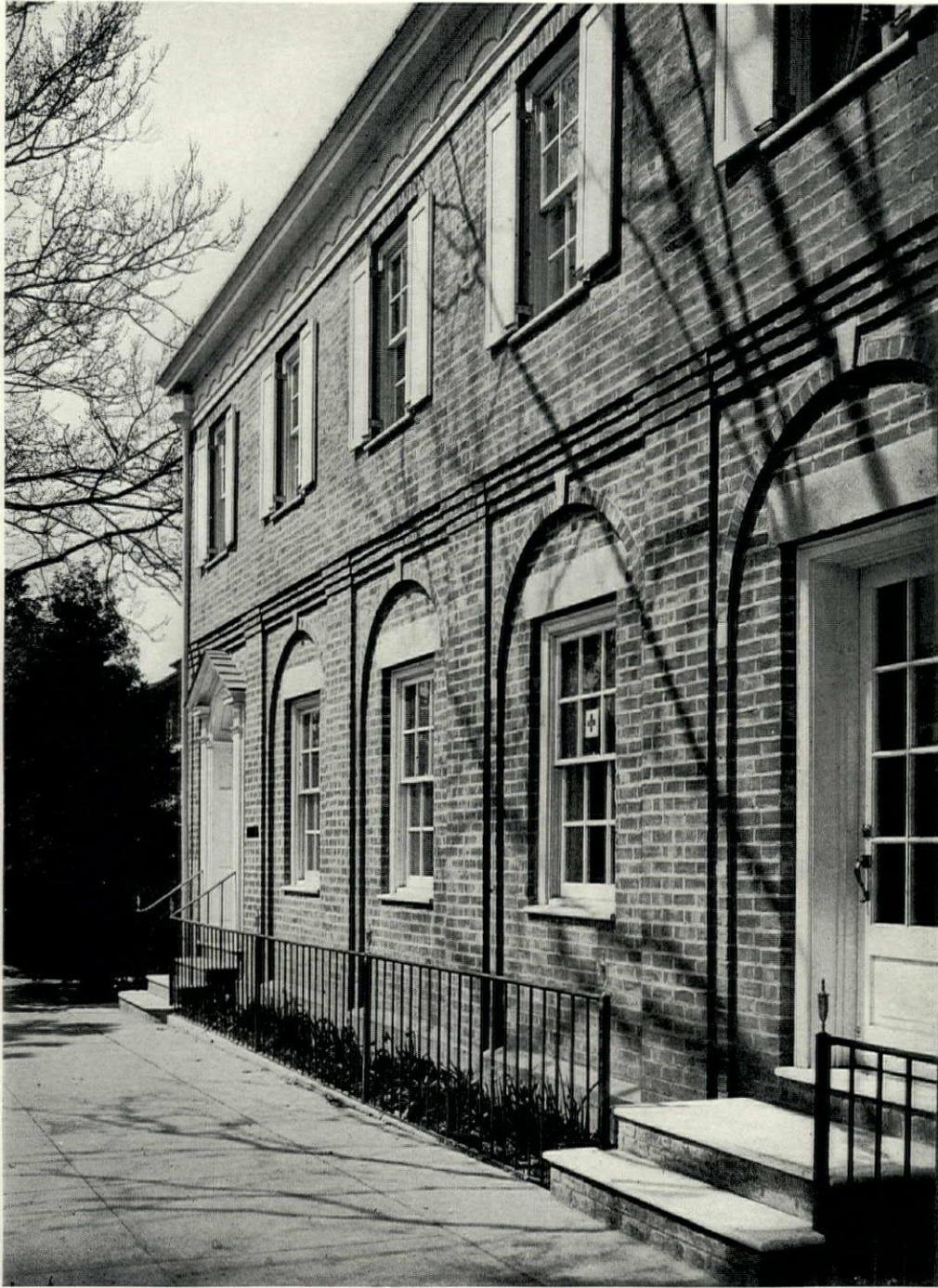
OFFICE BUILDING OF DR. W. C. MUDGETT, SOUTHERN PINES, NORTH CAROLINA Aymar Embury II, Architect
