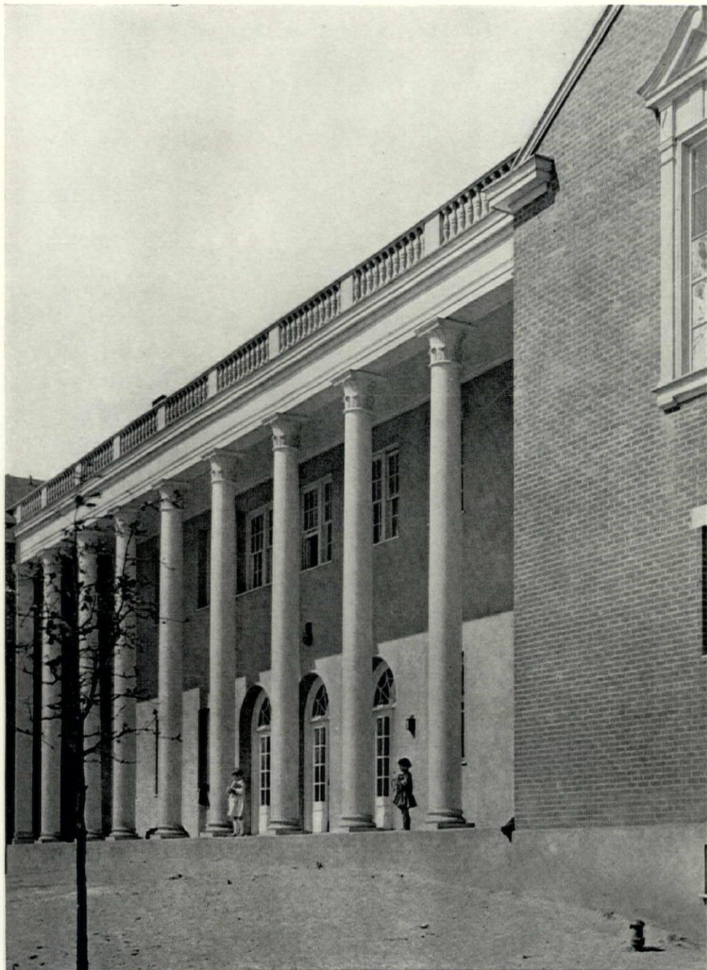
Detail of Portico THE ABERDEEN PUBLIC SCHOOL, ABERDEEN, NORTH CAROLINA Aymar Embury II, Architect
