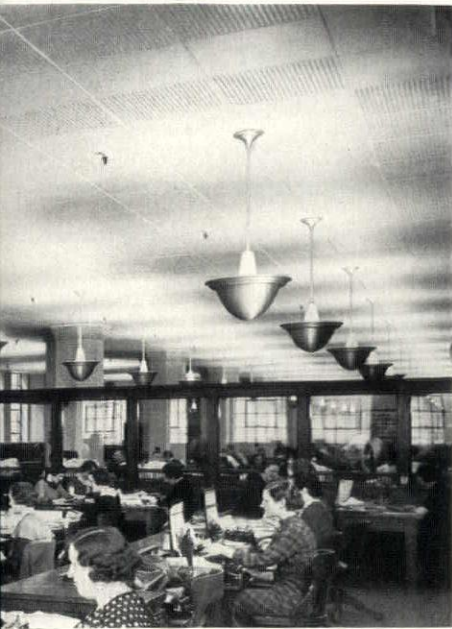
Tashjian ceiling with 900,000 air inlets
