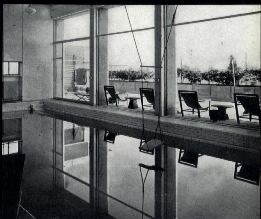
2 CRYSTAL HOUSE, CHICAGO. GEORGE F. KECK AND LELAND T. ATWOOD, ARCHITECTS. EXTERIOR WALLS ENTIRELY OF GLASS, ADJUSTABLE BLINDS TO CONTROL LIGHT. THERE ARE LARGE WOOD VENEER PANELS.
