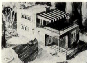
68 HACO SYSTEM—CONCRETE UNITS ON STEEL
