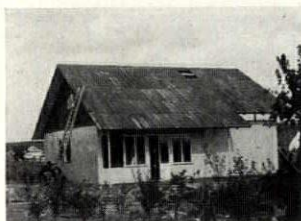
70 KLETZIN SYSTEM—INSULATED STEEL PANELS
