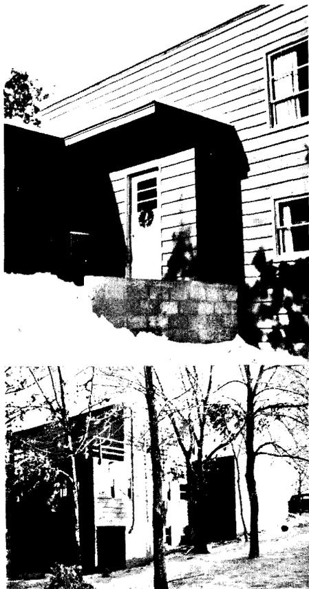
This residence was designed to house three occupants and one maid, with all bedrooms on what counts as the first floor. Because of the slope of the lot, nine feet from front to back of house, evident in lower view, the first floor in front becomes second floor in the rear. The ground floor is given over to recreation and laundry rooms, with space for the heating system. The simplicity shown in the design of the entrance is maintained throughout.
