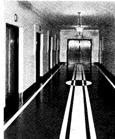
Elevator lobby, third floor, is 12 by 5 with a linoleum floor in terra cotta, and black. Base and dado are marble; and ceiling, plaster. Lighting is furnished by 3 semi-indirect fixtures.
