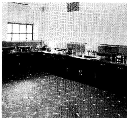
Kitchen floor and base are tile; walls and ceiling are of acoustic plaster; lighting direct, diffused. Equipment includes hot plates, toasters, sinks, refrigerators, incinerator, dishwasher, cabinets, and glass and plate tables.
