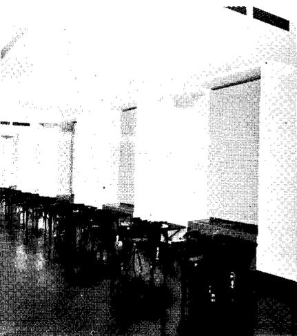
Waiting space for duplicating machine space. These have well as ceilings acoustically treated, using "Acousti-Celotex" perforated plaster. Floor is linoleum; base, slate; and lighting is direct.
