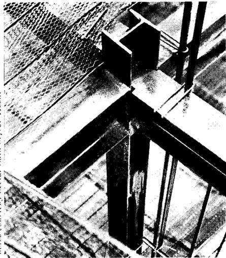
Lurie system (Metal Lath Mfrs.' Assn.) uses widely spaced steel frame, and metal lath supported on  $\frac{3}{4}$ -in. channels. Exterior walls consist of 2 in. of Gunite, an air space, an inside skin of plaster on metal lath. For floors and roofs see pages 89, 92.
