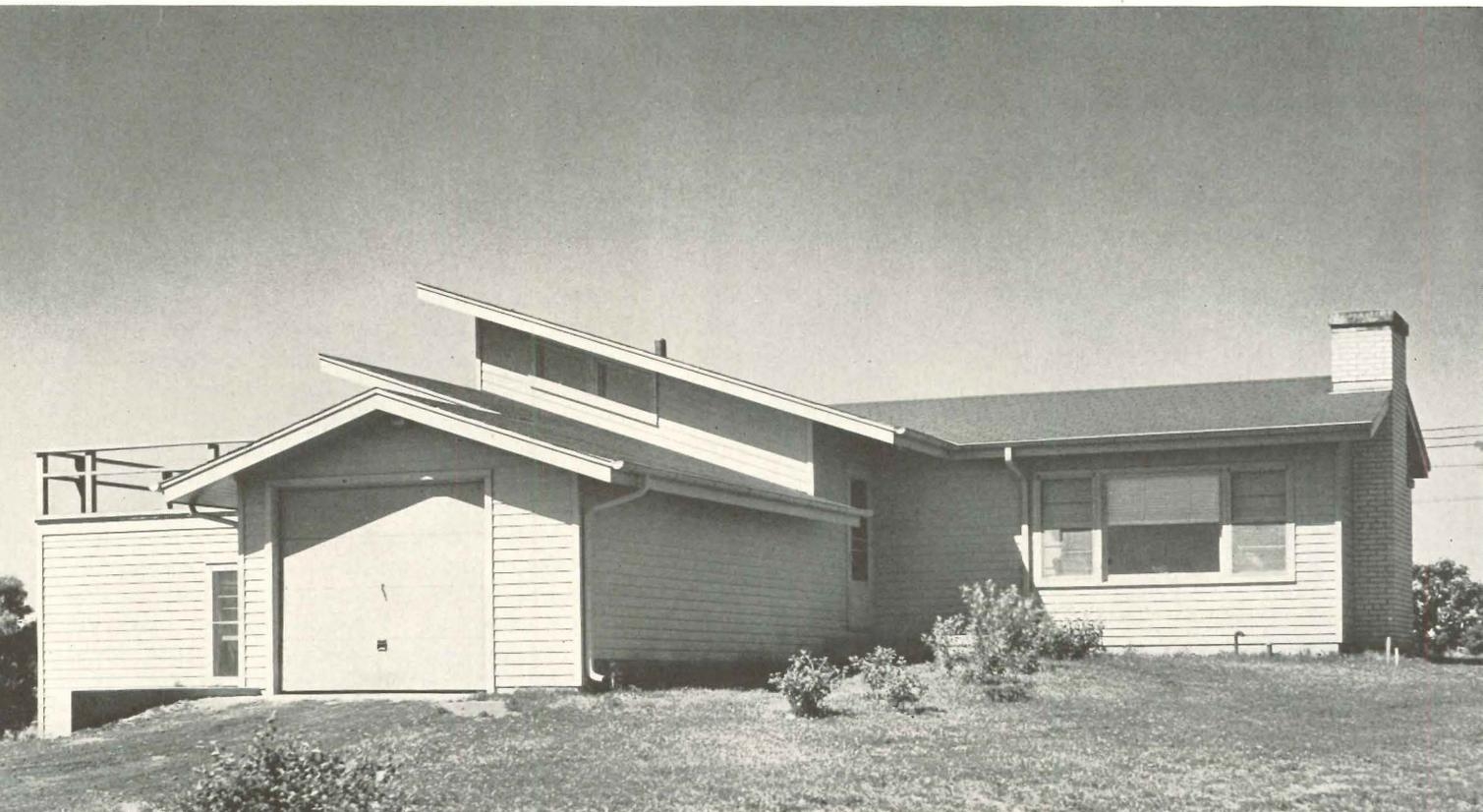
space now used as a sun deck; their addition will represent a completion of the exterior design. The exterior walls are painted sand color; shingles are blue black. Front and rear doors, garage door, and overhang soffits are painted sumac red. Interior walls are of plaster, painted in light colors.
