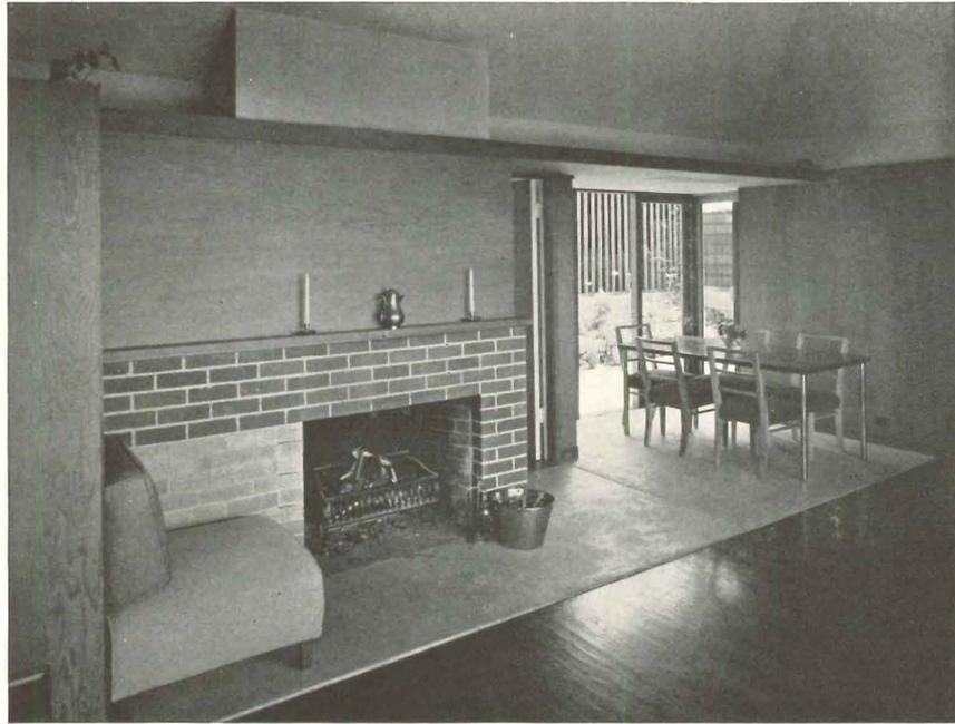
Omission of a partition between living room and dining alcove adds to the spaciousness of the area. Walls are redwood plywood, untreated; hearth is concrete.
