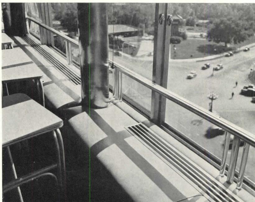
WINDOW DETAIL: remaining portion of parapet wall is capped with a 10-in. channel to which are attached the window tracks, made of aluminum channels and angles. Two out of each three windows slide horizontally. All are weatherstripped with refrigerator gaskets, and have concentric sash locks to strengthen their frames against wind pressure when closed
