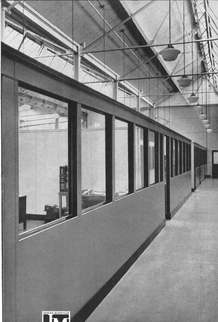
**YOU DON'T HAVE TO DELAY** your client—or specify makeshift materials—even when he wants a plant office put up *practically overnight!* Just specify J-M Transite Walls. These modern movable partitions go up fast—and long life with low maintenance is assured by their asbestos-cement composition. Check these advantages:
