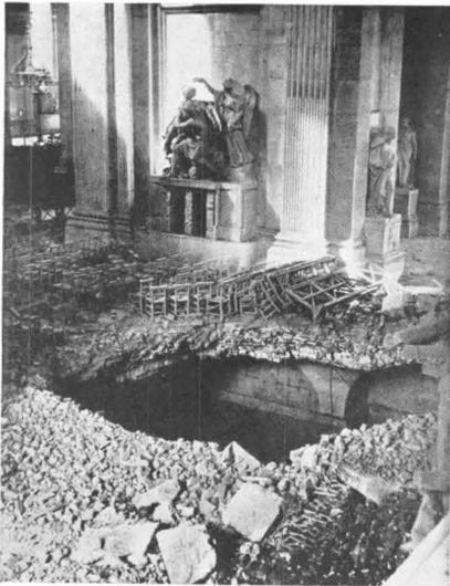
St. Paul's Cathedral has been hit twice by high explosive bombs. This view shows the north transept, where the debris caused the church floor to collapse into the crypt. Neither direct hit has interfered with the stability of the structure as a whole. Photograph from "The Bombed Buildings of Britain"
