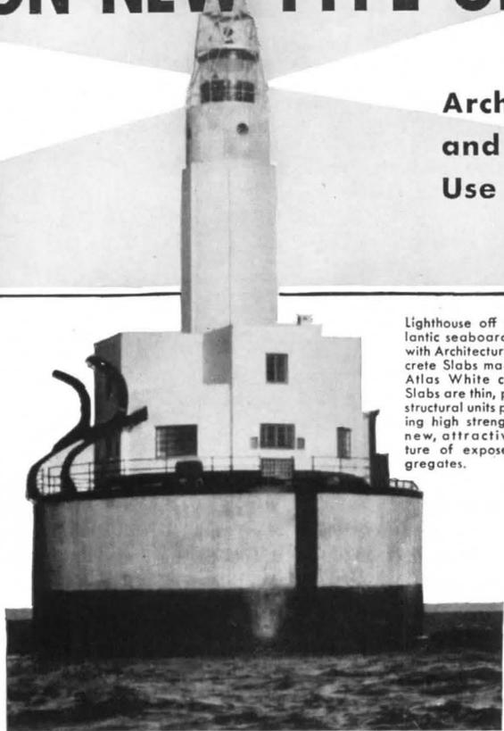
Lighthouse off the Atlantic seaboard faced with Architectural Concrete Slabs made with Atlas White cement. Slabs are thin, precast, structural units possessing high strength and new, attractive texture of exposed aggregates.
