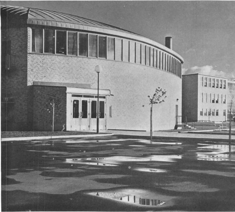
Left, exterior of the auditorium building from the north; domestic science buildings and laboratories at right. Continuous bank of windows lights the auditorium from above the topmost tier of auditorium seats. The double brick wall has heating pipes between and is open at the top. Ducts for air conditioning are over the stage (see page 48)
