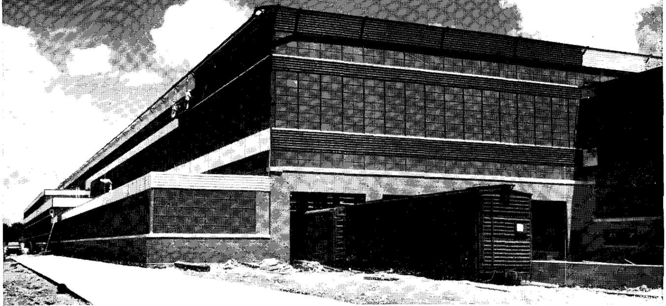
**Far out of practical range** of enemy bombers, a new Midwestern plant for the construction of submarine diesel engines is now in full operation. Noteworthy in this 300,720-sq. ft. plant is the provision made for daytime workers to work in clear, natural light. Over 60 per cent of the entire outer surface of the building, including the roof, is glass. Abundant sunlight floods the interior, making every department "clear as day," and thus stepping up production efficiency.
