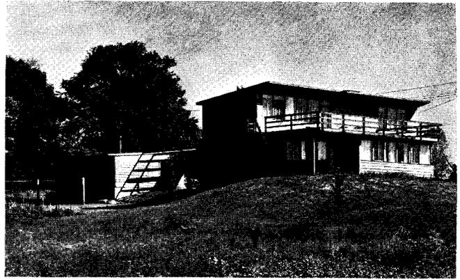
Full natural ventilation is achieved by openings between roof beams. Extension of the deck provides an opening at first floor ceiling; opening in living room ceiling at rear aids circulation
