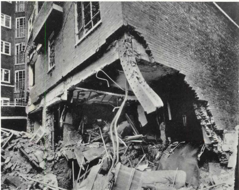
**1.** Steel-framed structures have the ability to withstand severe punishment from bombing without disintegrating as is the case with plain masonry structures.
