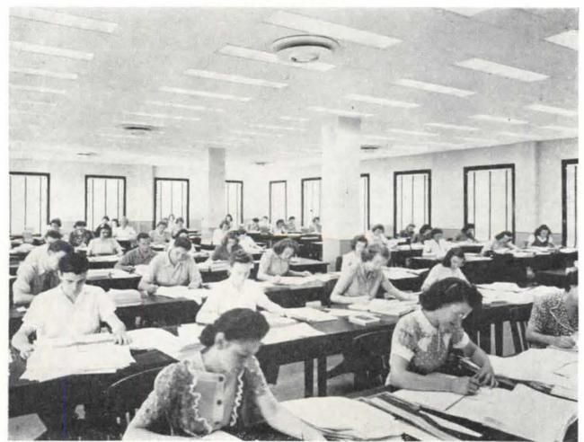
Figure 4: Brightness-contrast between lighting units and ceiling is low; glare is minimized. Work sheets happen to be large, thus surroundings of the task are bright, and seeing conditions good
