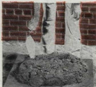
Mix a batch of 1-3 Brixment mortar (above) and a batch of 50-50 cement-lime mortar made with the same proportion of sand (below). Get any competent bricklayer to test them on the board—to spread them on the wall—to lay up a few brick with each of the two mortars. Then ask him which has the best workability!
