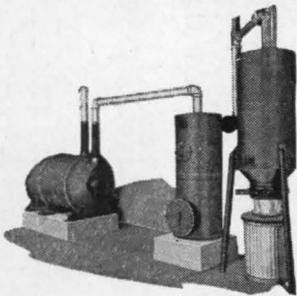
The vacuum producer and dirt container are located in the basement. Piping connects to convenient inlets all over the building.
