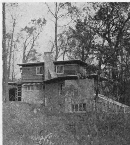
*The living-room end of the wing-nut plan utilizes natural contours to put greenhouse (on south wall) at basement level, and to give maid's room, bath full window height*
