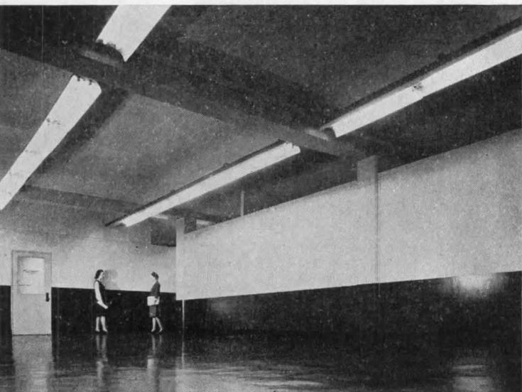
reinforced concrete. And putting a reinforced concrete roof over 40 by 40-ft. bays was by no means ordinary construction.
