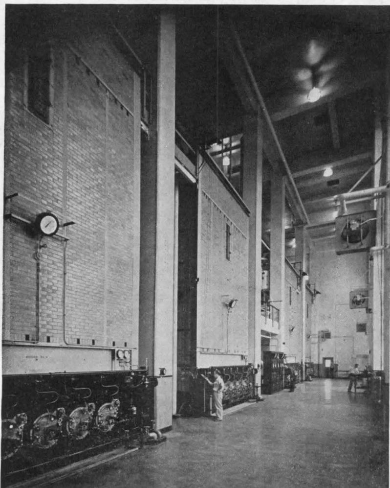
*Four huge boilers, each with a capacity of 100,000 lb. of steam per hour, supply steam at 175 psi. Boilers are oil-fired, can burn refuse oil if required; two are also connected to rubbish incinerators*
