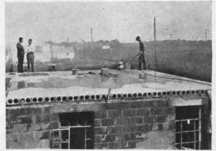
*Speedy installation is one feature of a new precast, hollow-cast roof slab*
