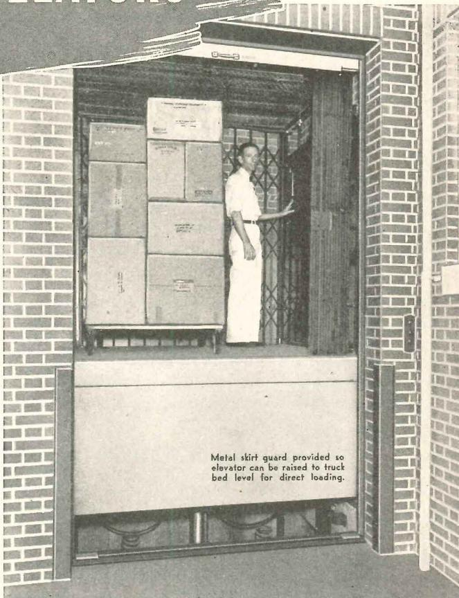
Metal skirt guard provided so elevator can be raised to truck bed level for direct loading.
