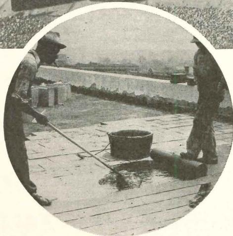
This re-roofing job includes *permanent* insulation with PC Foamglas. On new construction and on modernization projects on all sorts of plants, PC Foamglas Insulation has licked the toughest jobs. An impervious, inorganic, cellular material, PC Foamglas, retains its insulating value—*indefinitely*.
