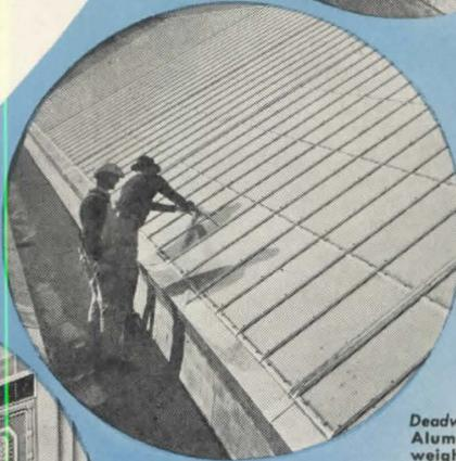
Deadweight is eliminated here. Aluminum skylights are light in weight and provide excellent weather-resisting qualities.
