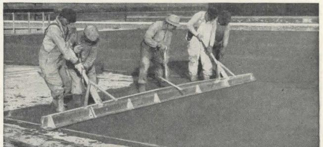
• Screeding Zonolite Insulating Concrete roof fill over concrete slab. Easily formed into saddles and cants for proper drainage.
