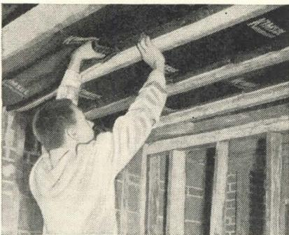
Installing light, flexible KIMSUL\* in a CAPITOL PROPERTIES, INC. home. It is easy—just cut KIMSUL to desired length, expand it, and staple to ceiling joists.
