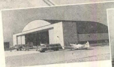
170' x 120' hangar at Hagerstown, Maryland, designed by Albert Kahn, Associated Architects and Engineers. Roof supported by 170' wide Unit glued-laminated arches.
