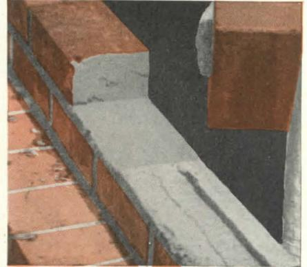
Then the excess mortar will fill the furrow and insure full bed joints.
