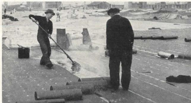
**THE UNIFORM** texture and thickness of Barrett Specification\* Felt are appreciated by experienced architects and contractors. Accurately spaced longitudinal guide lines marked on the felt are an aid to quick and accurate application.
