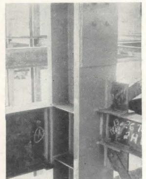
**Fig. 3. Corner of elevator opening showing only place where cross-bracing is employed.**
