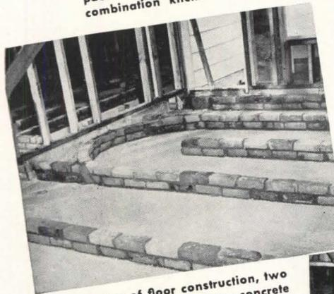
Beginning of floor construction, two tiers of bricks are laid on concrete slab to form heat distribution ducts 5½" deep.
