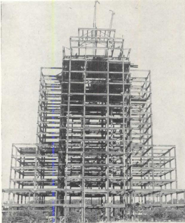
**Fig. 1. All-welded structure of Hermann Professional Building.**
