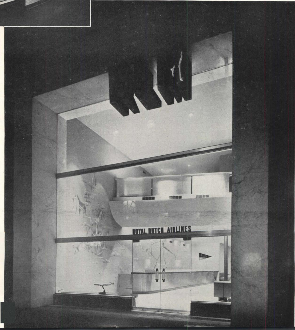
Much of the striking effect of the design was due to the simple, uninterrupted width of the plate glass panels. The upper lights, approximately 20 by 7 ft., each, are of  $\frac{3}{8}$ -in. glass, about the largest plate glass made in that thickness. The lower panel is of  $\frac{3}{4}$ -in. plate glass and the doors are of herculite of the same thickness, hung on self-closing door hinges to eliminate the necessity for a frame which would interrupt the wide expanse
