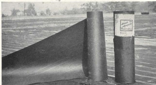
**COMPANION TO** Barrett Specification\* Pitch is Barrett Specification\* Felt—the *only* felt good enough for a Barrett Specification\* Roof. It is made from carefully selected and fabricated stock and special coal-tar saturant to meet rigid manufacturing standards.
