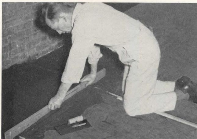
FIG. 3—Floor fill is mixed and applied to the floor like concrete topping. Wood screeds control thickness of the fill which is leveled with a straightedge. The surface of the fill is smoothed with a trowel and, where necessary, it can be troweled to a featheredge.
