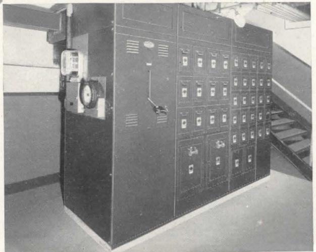
CAPACITIES: 30 to 1200 amps., 250 volts, AC or DC; and 575 volts, AC, in 2, 3 and 4 poles. See your nearest
