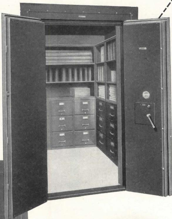
Herring-Hall-Marvin insulated flat sill *double door* vault entrances give you the choice of any degree of certified fire protection . . . plus the extra convenience of a wider entrance, full 42" clearance for easier movement of record buses and trucks.
