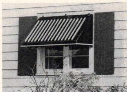
Awning louvers, adjusted by a control arm, permit any degree of light and ventilation
