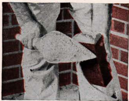
Method 1. Plenty of mortar should be thrown on the end of the brick to be placed.
