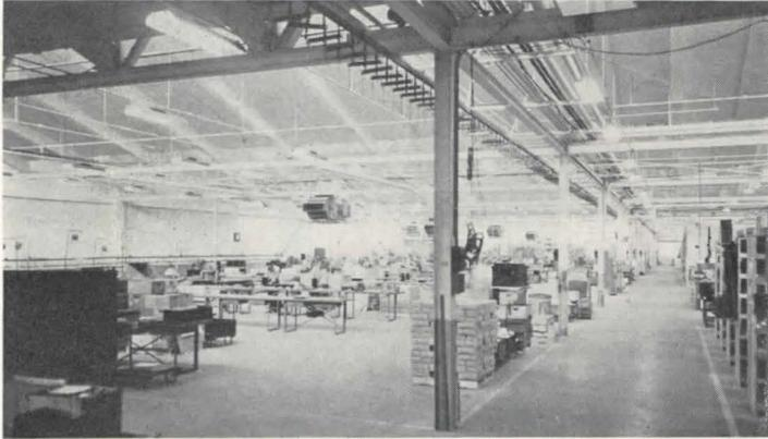
*To eliminate much grading, the factory floor was given a mild slope—1.11 per cent—which is really imperceptible. The material flow, however, is arranged so that trucking operations take advantage of the grade*
