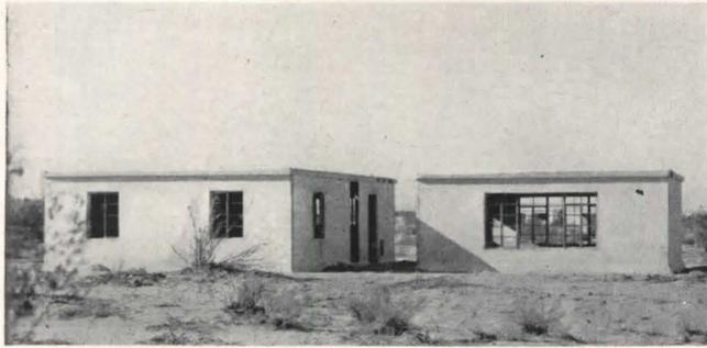
Left: two sizes of house forms are used for each double unit at Muroc, the two delivered to the site by Tournalayer and set 7 ft. apart; a conventionally constructed corridor joins them. Above: an overhanging eave "dresses up" a duplex unit
