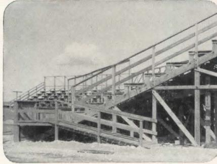
1. Ground moisture and rain held in joints etc., of outdoor structures.
