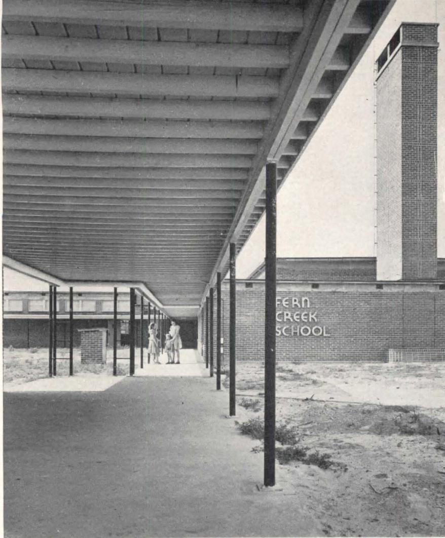
Cavity wall construction uses 4 in. of red brick for outside face, 3 in. air space, 4 in. of brick and concrete block in interior. (Detail shows openings left for ventilation.) Cost of bar joists only slightly exceeded local lumber cost. Ceilings are of acoustical tile on wooden furring; walls of soft pine yield tack space. Plastering omitted except in toilet rooms and the kitchen, where it is used in conjunction with ceramic tile
