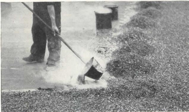
**SPECIAL FEATURE** of the Barrett Specification\* Roof is the gravel or slag surface. The built-up layers of pitch and felt are topped by a thick *pouring* of pitch to *anchor* the gravel or slag thus providing armored protection for the waterproofing membrane below.
