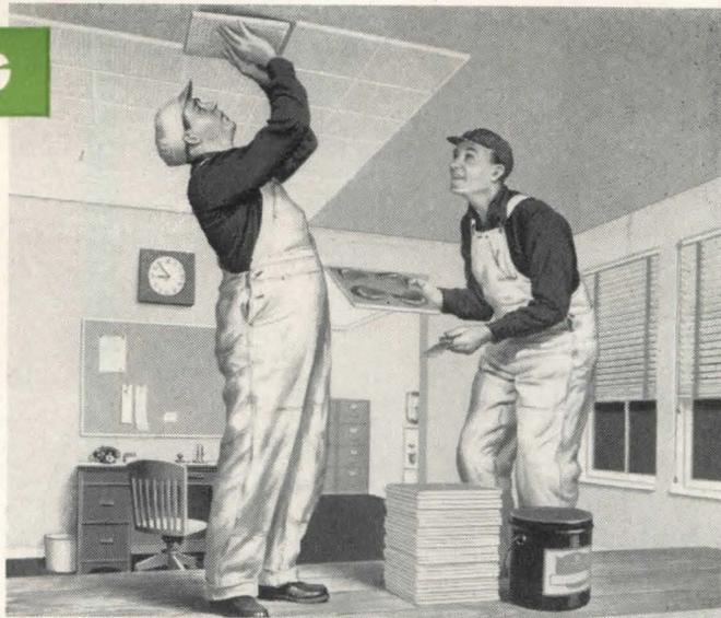
A factor of importance in sound conditioning is selection of an adhesive that will hold acoustical ceiling tiles in place permanently. Results of an eight-year test on twelve brands of acoustical cement reveal marked variations in characteristics, and indicate that architects should specify not only the acoustical material but also the proper cement to keep it in place.
