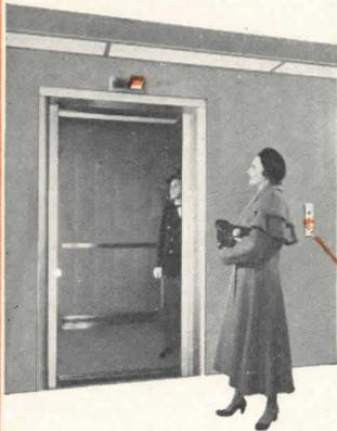
**FOR THE PASSENGERS** —it's a 'touch' of magic. It's the newest way to call an elevator. How? By simply *touching*, not pushing, a plastic arrow in the landing fixture. What happens? The electronic 'touch' button lights up. A soft-toned gong announces an approaching elevator as the overhead lantern lights up. The passenger steps toward the entrance, the doors open—and she's on her way. How's it done? With a magic brain—the *electronic panel in the control room*—as pictured below.
