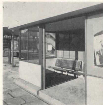
of railway work. The wall required, for example, an impervious, easily cleaned and attractive finish above flow level; below flow level, a hard surface to resist damage from barrows was essential. It was desirable to obtain certain levels of insulation from the point of view of comfort and economy in heating. It was also desirable that the wall thickness should be cut down to a minimum.
