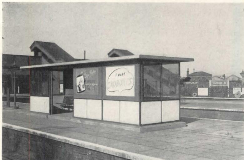
This small island building—also prefabricated of enameled iron panels—serves as a sheltered waiting room, with neatly designed wood-slat benches inside
