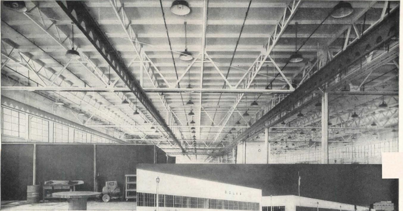
82,535 sq. ft. of Cemesto, clipped to steel beams, provides insulation, light-reflecting interior finish, and great strength with light weight — applied as structural roof deck on the Solar Aircraft Company's new plant, San Diego, California.
