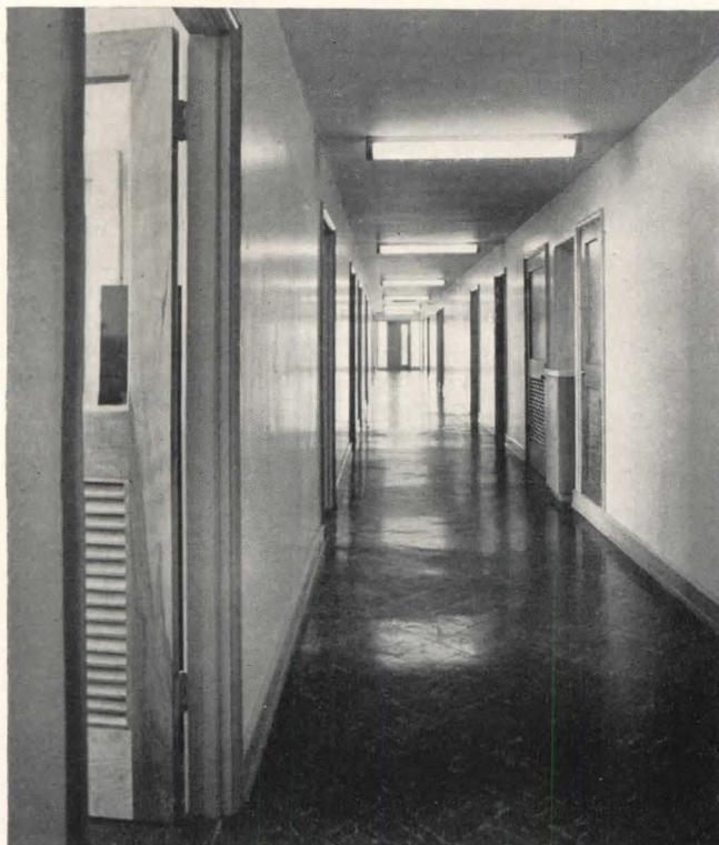
This corridor photograph could have been taken in either of the two office buildings, as both interiors are identical. Ceilings are furred down for air conditioning ducts; floors, asphalt tile
