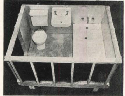
*Only connections necessary to this integral, prefabricated bathroom unit are the hot and cold water, waste and vent*
