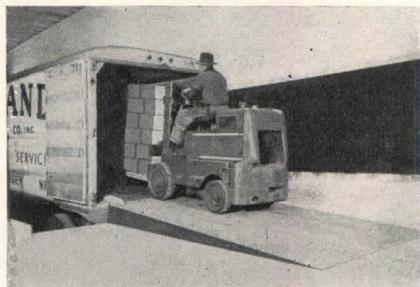
Trucks and trailers loaded without steel plates or bridge ramps by application of a hydraulic loading ramp, the *Leva-Dock*
