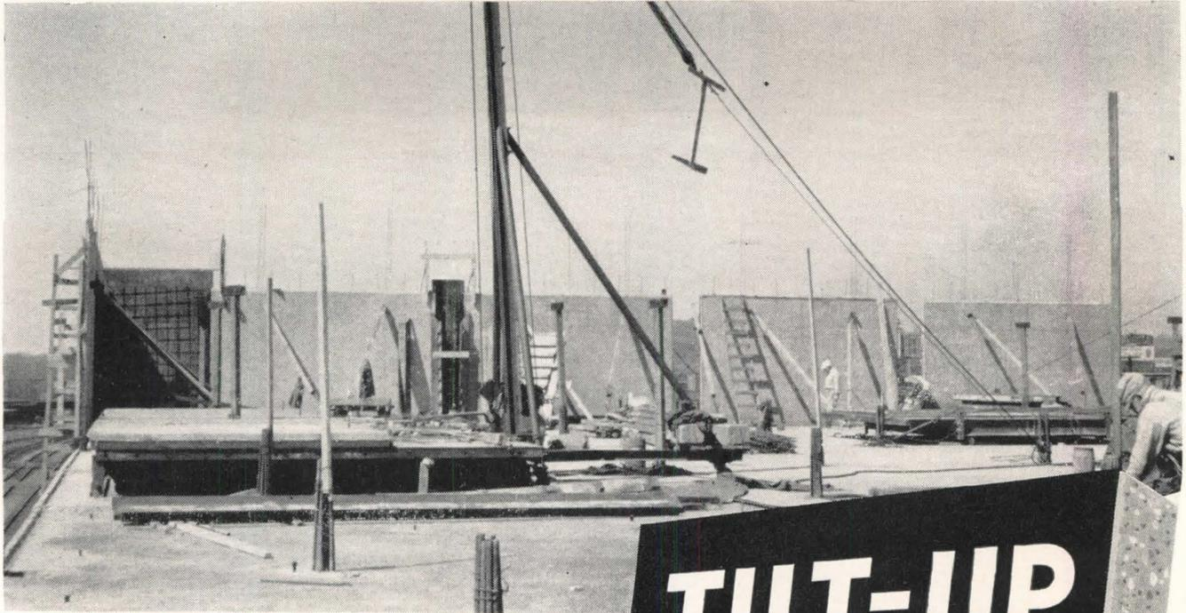
**TILT-UP**, the fast, economical method of concrete construction was used in building the new warehouse of the Merchants Transfer & Storage Company in Des Moines, Iowa—a 3-story structure 95x188 ft. in size.
