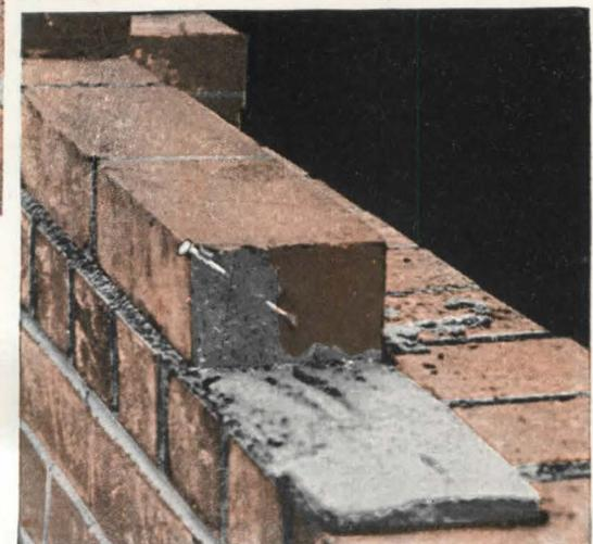
Water entering through the nail holes may travel through connecting voids and find an opening to the inside of the building.
