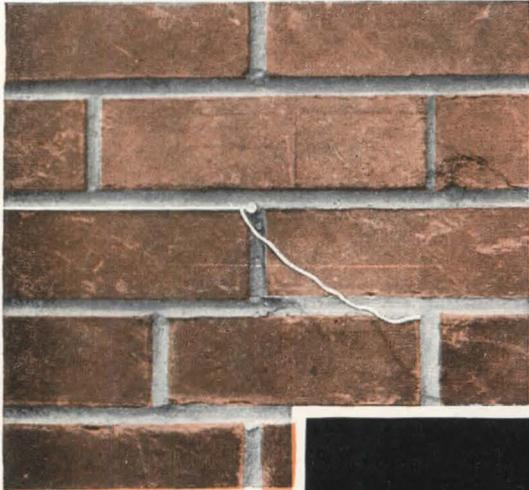
When a nail or line pin is used, the hole should be plugged with mortar as soon as the nail is removed.
