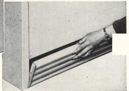
**NEW SNAP-IN GRILLE!** Completes striking appearance of *Modine* Convector. An optional feature you can add now or later. Snaps in or out of place without tools. Affords quick access for cleaning beneath cabinet.
