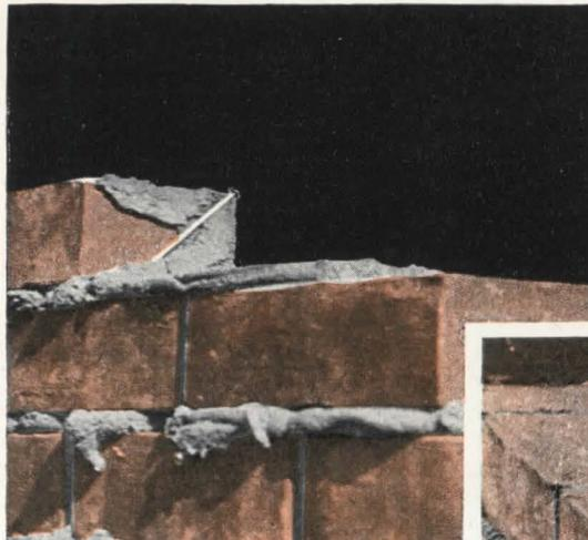
Nail holes frequently connect with voids in the head joints which in turn connect with unfilled furrows in the bed joint.
