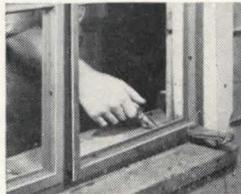
**B** After erecting, before glazing, test fit of each ventilator by pushing it closed. Ventilator top should touch first while bottom extends about 1/2" from frame. Later, when hardware is installed, underscreen operator will draw in bottom of ventilator.
