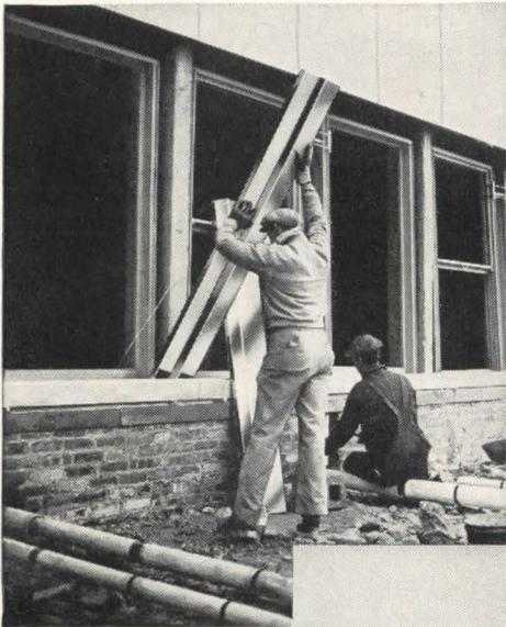
*Mullion is screwed to an angle, which is an integral part of the window frame, by stainless steel self-tapping screws.*
