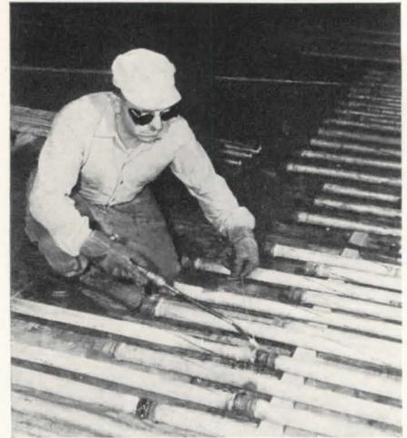
Operator applies silver alloy to braze threadless joint with piping in place
