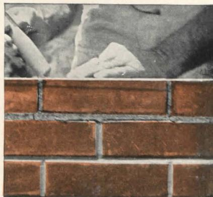
Brick should be laid true to the line, when originally placed. If any delay occurs before they are tapped into place, the bond will be broken and a crack will result. Realignment of a brick should never be attempted after a higher or following course has been laid.
