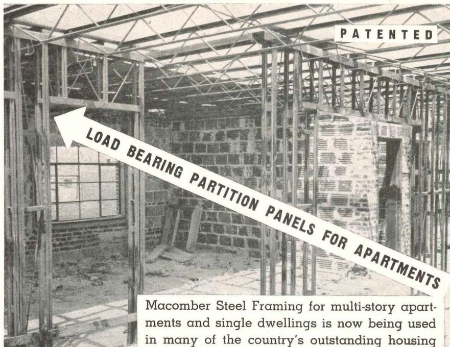
Macomber Steel Framing for multi-story apartments and single dwellings is now being used in many of the country's outstanding housing projects. These nailable steel framing units are fabricated to specified loadings and for structural layouts of similar design.
