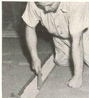
**2. Almost invisible seaming!** *Cushionlok* has a special Trim-easy edge which strips off, leaving neat edges that meet almost invisibly. *Cushionlok* is then cemented to the floor.
