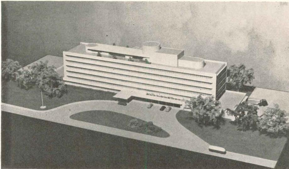
light, also horizontal. Moreover, the continual dampness virtually made a basement impossible; this accounts for the extended first floor for mechanical equipment (penthouse superstructure houses cooling tower and fan rooms).
