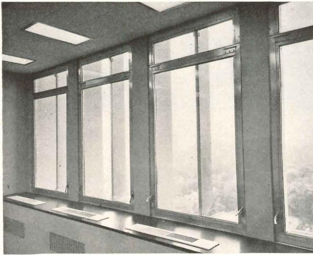
Sunshades on the north side (left) are fixed in vertical position half way between stone mullions — they protect against early morning and late afternoon sunlight. Horizontal shades (above) rotate through 180° — those for each window can be controlled separately, but all for that window are controlled in unison
