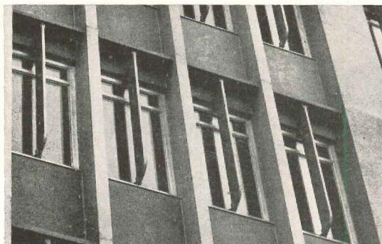
The Sealuxe Thermo Windows on the north exposure have a fixed center vertical shade that prevents the heat waves of the late summer sun from striking the windows.
