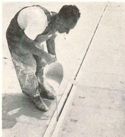
Left: lightweight, insulating roof tile is transported to work areas by wheelbarrow and then laid over structural steel members. Below: joints are grouted with mix of gauging plaster, vermiculite and water
