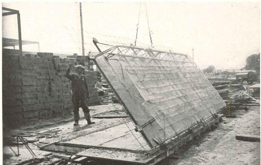
building was constructed of reinforced concrete right on the grade. The second floor was originally designed to be of reinforced concrete slab and beam construction. In order to try out the prefabricated panel system, the owners of the building agreed to allow it to be used in place of the construction originally specified for the second floor, on condition that the proposed floor system should not cost any more than that originally specified.
