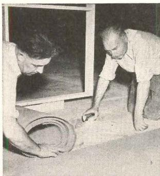
**1. Cushionlok goes down on bare concrete.** Can be laid, with no time-taking workroom tasks, on concrete, wood or plywood. Requires no cushion—the cushion is *part* of *Cushionlok*.
