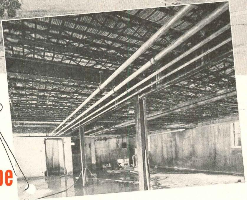
In this group of ten cottages and a recreational building, the designers recognized the importance of building for *durability*, as a hedge against high maintenance costs. The hot water lines, the cold water lines, the vents and drainage lines under 2-inches, and the condensate returns in the heating tunnel were all specified "wrought iron". Byers Wrought Iron pipe was installed. Of equal importance—*wrought iron nipples* were used in all these lines, so no "weak links" would be present.
