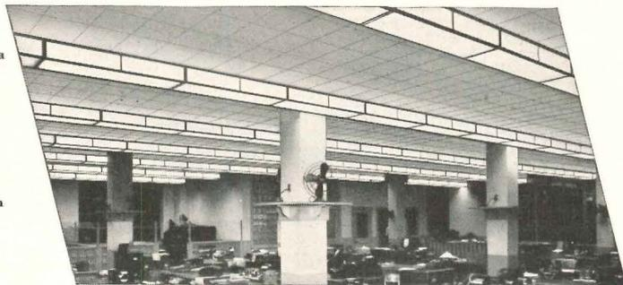
● Individual or continuous runs provide flexibility of arrangement to fit any ceiling light pattern desired.
