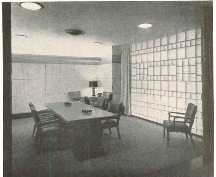
*In the large executive-conference room, the front wall of glass block achieves an interesting textural pattern, as well as admitting maximum daylight while preserving the privacy of the room and shielding the occupants against both the noise and the distractions of the sidewalk just outside. Note the flexible partition*
