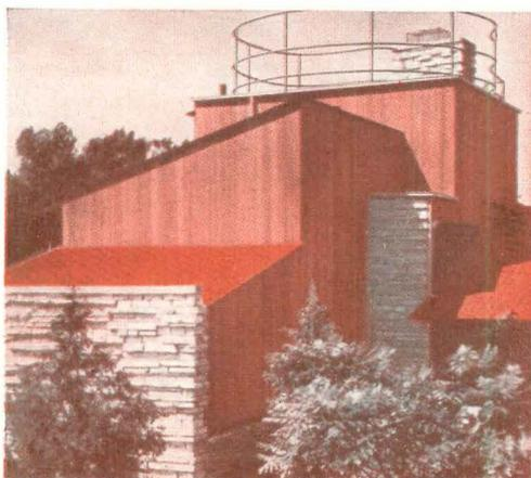
● Designed by George Fred Keck, William Keck, Architects, the house pictured was built in 1939 near Fish Creek in Door County, Wisconsin. Using local limestone, the house features Redwood siding and a heavy butt, dark red Asphalt Shingle. The wing above provides a third floor study and captures a view of Green Bay. Note that in 1939, with all roofing materials in plentiful supply, Asphalt was both a design and functional choice.
