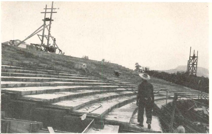
Left, grade-level entrance to ramps leading to second-level seating and boxes. Above, second level partially completed; formwork for a vomitory in the foreground
