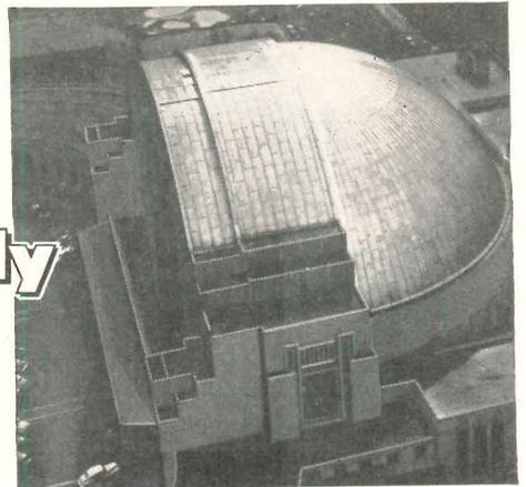
Overly's Goodwin Batten Type aluminum roofing installed on the huge 150 foot dome of the Cincinnati Union Terminal.
