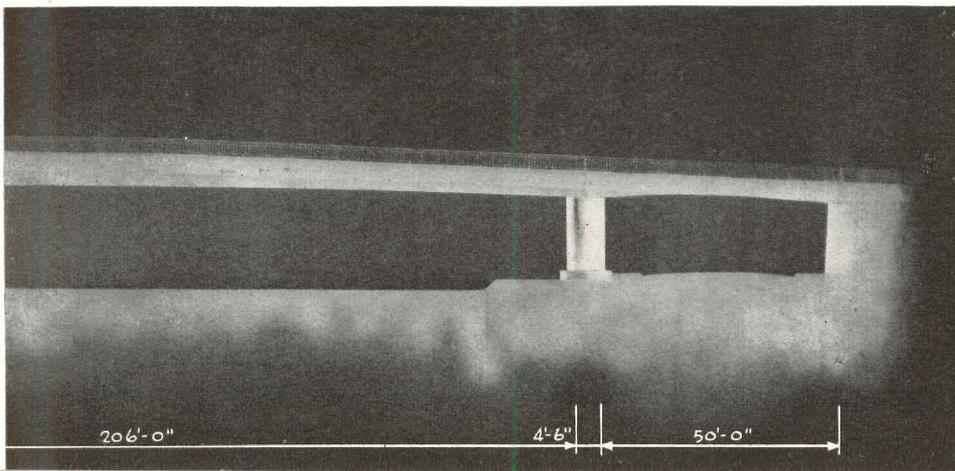
1. Bridge over Marne at Luzancy, France, span 182 ft. Designed by Freyssinet, the bridge has depth to span ratio of 1 to 45. 2, 3. Another Freyssinet bridge, this one at Esbly, has 240 ft. span. These bridges were assembled from precast sections. 4. First continuous bridge to be built with prestressed concrete, going up over Meuse at Sclayn, Belgium; supervising the project is Prof. Gustave Magnel. Shape at the center pier is completely functional
