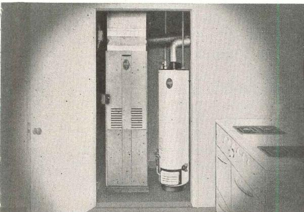
1,223 APARTMENTS at Drexelbrook are equipped with Bryant Personalized Heating. Shown are the Bryant Model VS-304 Winter Air Conditioner and Bryant Red Seal Automatic Gas Water Heater in closet installation. 50 community laundries also are equipped with Bryant Water Heaters.
