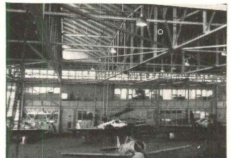
↑ This airplane repair shop is protected by the Grinnell MULTITROL System, which employs a release device actuated by the *rate of rise* of the temperature, rather than by the *degree* of temperature. This is one of several Grinnell Fire Protection Systems for special conditions and hazards.
