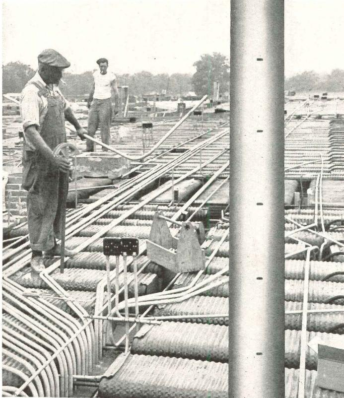
*Typical of countless ELECTRUNITE E.M.T. "in concrete" installations, is this large midwest apartment project. Light weight, ease of handling and limited space requirements make ELECTRUNITE E.M.T. ideally suited for concrete construction.*
