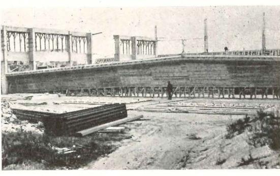
16. Hangar at Melsbroek, airport of Brussels; one prestressed beam carries load of 3,500 tons. 17, 18. Use of 168 ft. beams of prestressed concrete allowed a clear height of 32 ft. from floor to beams
