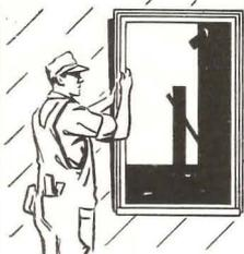
**ALL INSTALLATION MEMBERS OF TOXIC-TREATED WOOD... WATER-PROOF FELT WEATHER STRIPPING ASSURES WEATHER-TIGHT CLOSURE—EASE OF OPERATION—NO RATTLING... SIMPLE INSTALLATION CUTS FIELD COSTS—Simply insert wood surround into window opening and nail in place. Glass and screen panels may be inserted when desired...**
