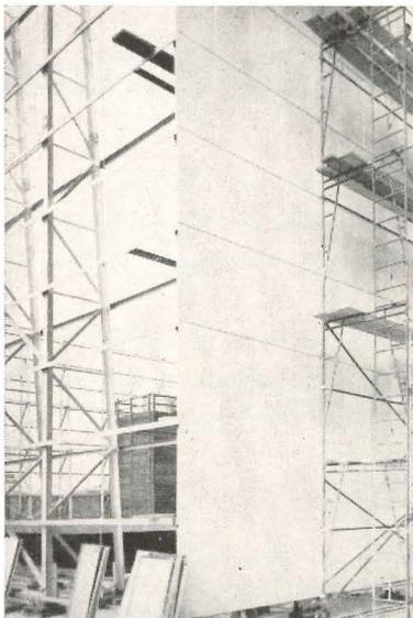
Topping this new magnificent building is an installation of over 24,500 square feet of Seaporcel Porcelain Enamel . . . yes, virtually 30 tons of this mechanically fastened material of permanence and beauty.
