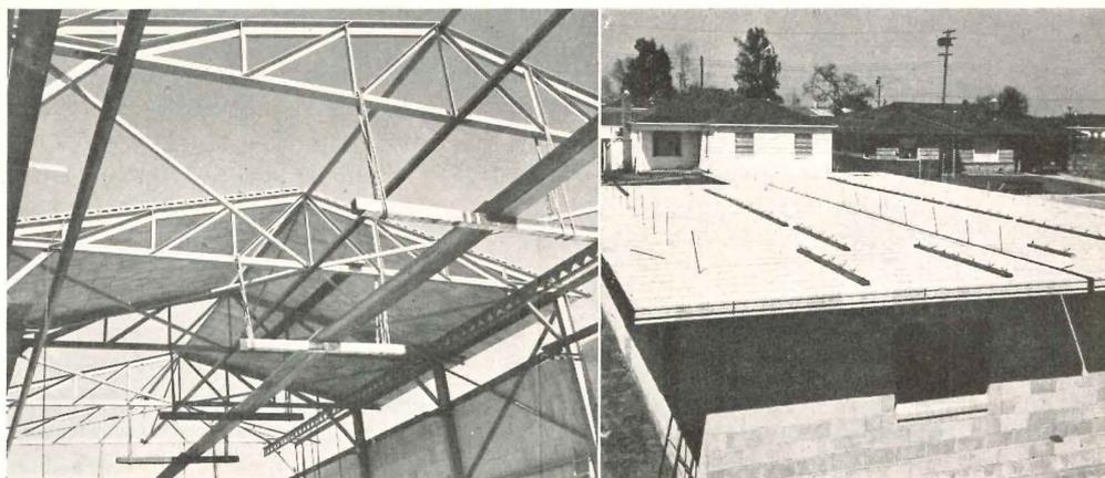
At right, above: *Strestcrete* roof slab on home in Sacramento, where 2000 ft. of roof were laid in 3½ hrs. Above, at left: roof trusses with *Strestcrete* roof slabs in place waiting to be grouted. Panels are lifted into place by use of a crane and attached to steel framework for welding. No purlins are used. For roof construction, slabs that span 32 ft. are reported to be practical. Slabs and panels are assembled to specified dimensions
