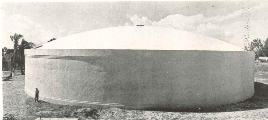
19. In manufacture of prestressed concrete tanks, machine stresses high strength wire by pulling it through a die as it is spiralled around the tank; the wire is later covered with gunite. 20. This prestressed water tank in Miami, Fla., has a diameter of 128 ft., depth of liquid 27 ft. 8 in., and capacity 2,700,000 gal.
