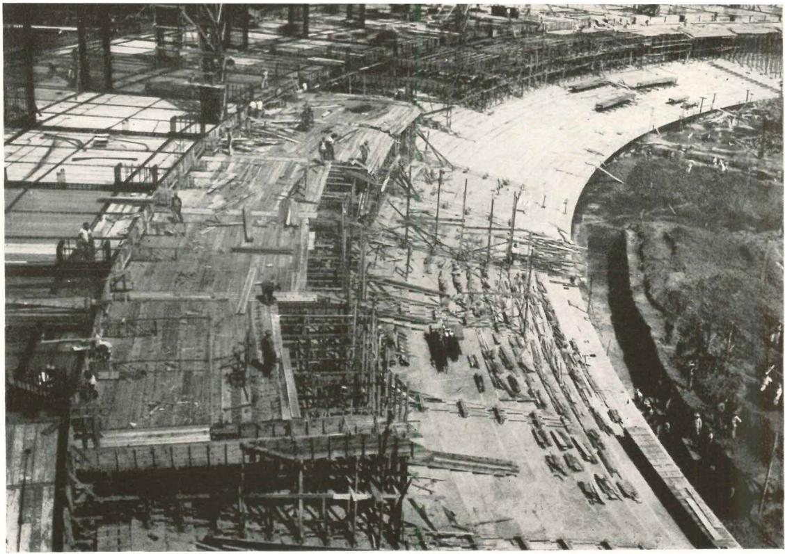
*Above, second level construction completed, forms under way for third, as of April 23, 1949. Across page, another view of second level; private boxes are at the rear of this level, between the columns which will support the third level. Below, panoramic view at same stage of construction, showing start of complex formwork to support a 65-ft. cantilever during pouring*
