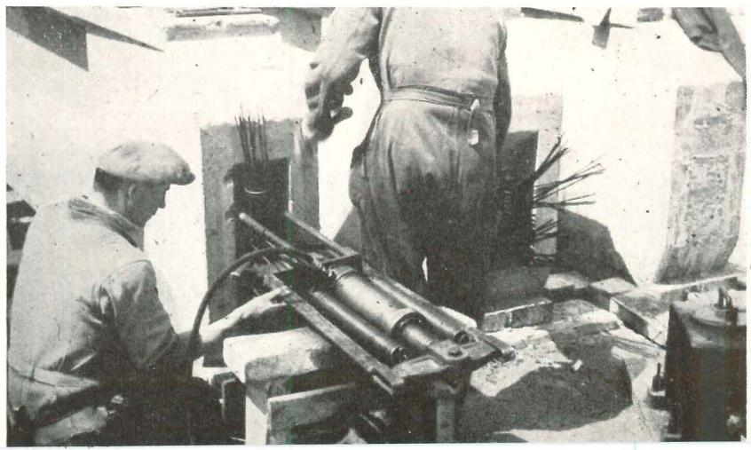
12, 13, 14, 15. Prestressing as done by the Belgian method. 12. End of girder before it is prestressed; cables are strung through beam after concrete is hard. 13. End of girder after wires have been tensioned by a hydraulic jack (14) and anchored by means of sandwich plates; pipes sticking out are for injecting grout after girder is prestressed
