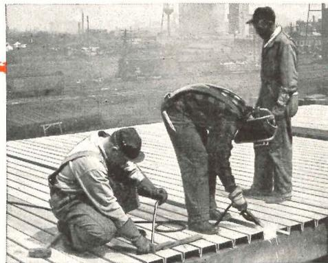
**WHEELING TRI-RIB ROOF DECK**
