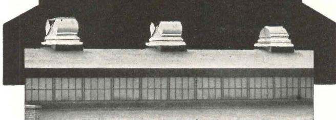
Where you have heat, smoke and fumes in concentrated quantities, it takes *power* to expel these elements fast enough to clear the atmosphere for greatest comfort. Swartwout Ject-O-Valve forces contaminated air outside before it spreads through workrooms—draws *fresh* air in from outer walls.
