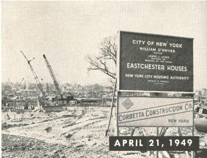
CONCRETING better than a floor a day, it took just 65 working days to erect superstructures of the ten units, 7 and 8 stories high, for Eastchester Houses—New York City Housing Authority's 874-apartment project, 950,000 sq. ft. floor area, in the Bronx.
