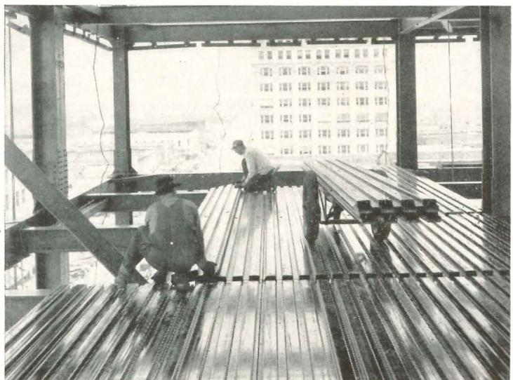
RIGHT. At the Commercial National Bank in Shreveport, La., (McKim, Mead & White, architects; S. G. Wiener, Asso. Archt.) Q-Floor is installed. It is welded directly to the beams over which light-weight concrete fill is placed to provide a level surface. The cells are available for the distribution of electrical and telephone wiring. Changes can be made quickly.
