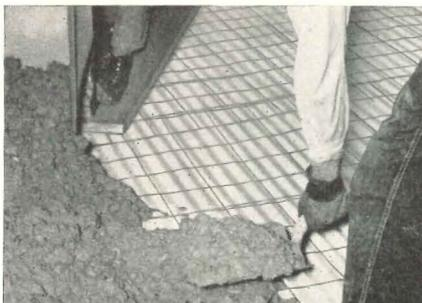
**2. ECONOMICAL**—Light high-strength — 100,000 psi—steel to take construction abuse. No sag or material waste, concrete placed and finished by common practice on firm stable CORRUFORM.
