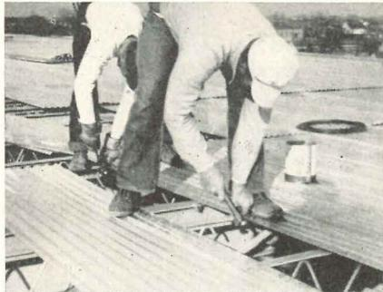
**1. SAFE**—Light rigid sheets and attachments easily placed. A secure form for trades and concrete. No stretch or side pull on joists, beams or walls.
