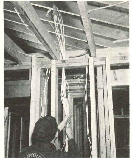
Remote control electrical system uses thin wires (above), has selector switch for 9 outlets (below)
