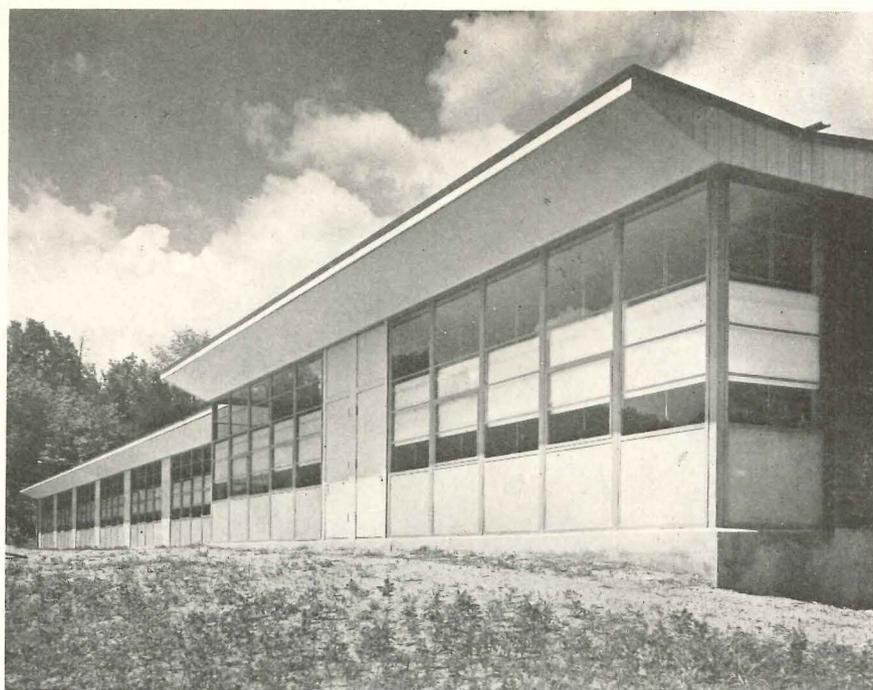
*The classrooms face south and have doors to the outside. Sheets formed of insulation between asbestos cement layers form the wall below steel windows*
