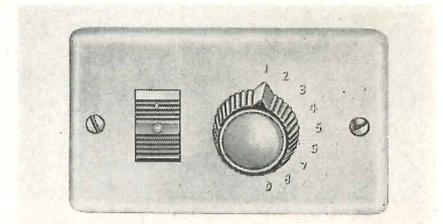
The system uses lightweight thermo-plastic remote-control wire, which can be stapled to joists, etc., and can be used where full voltage conduits cannot be readily installed. The 24 volt system can carry full rating of fluorescent lamp loads. *Master Selector Switches, GE3652*, control principal circuits. The unit is of the rotating type, with separate on and off switch, and controls one or all of 9 circuits. General Electric Co., Bridgeport 2, Conn.
