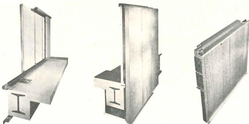
Illustrations from *Stainless Steel Curtain Walls — A Progress Report On Methods*: left, back and front of metal pan design combined with structural insulation; right, view of reinforcing-type textured steel facing, cast insulation
