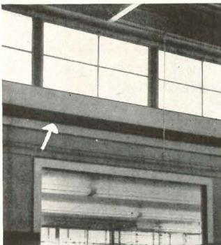
**LOW:** Vulcan two-high running full length of glass wall provides convection blanket of warm air for full protection of personnel.
