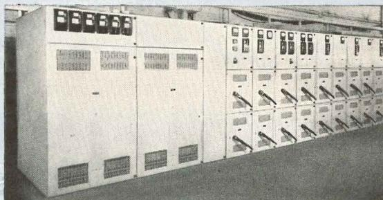
**THE MODERN WAY** . . . Westinghouse "Unitized", Low-Voltage Switchgear. Metal-enclosed air circuit breakers speed servicing . . . are interlocked for safety. All operations accomplished without exposing live parts.
