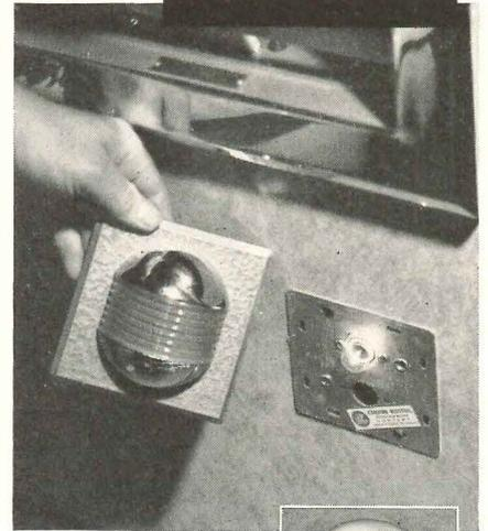
(Above) DNP-1 light used in residence, with face plate removed, showing construction of (2 gang) plaster ring box cover.
