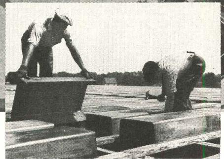
Labor of placing and removing steel-forms by skilled Ceco workmen is ordinarily included with the rental charge.
