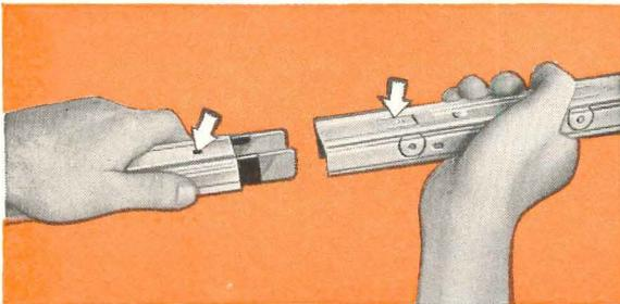
Duct sections are joined without tools, nuts or screws. Prefabricated and standardized in lengths from one to ten feet, they can be dismantled and reinstalled anytime, anywhere without scrapping a single part.
