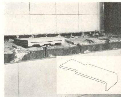
Wrought iron clips (detail at right) fasten ceramic tiles securely in place
