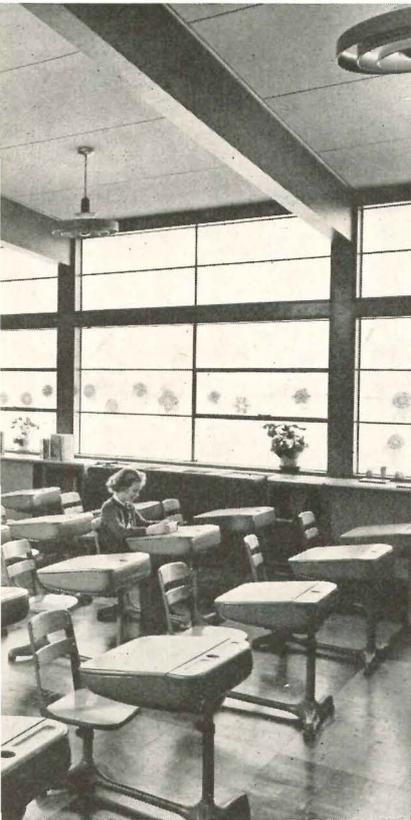
Note framing module based on steel sash and plywood sizes
