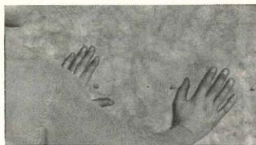
**3** Insulation is quickly installed by impaling it over studs.
