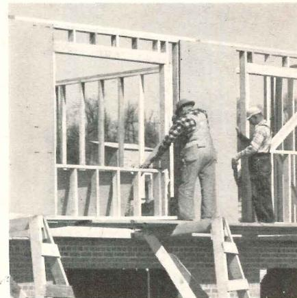
**Insulite Bildrite Sheathing** on exterior wall saved Sauers Construction Company hundreds of dollars on every Sibley Manor U because no corner bracing was required. BILDRITE has twice the bracing strength and insulation value of horizontally applied wood, yet applied cost is far less!
