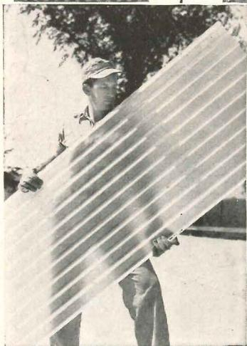
Resolite is shatterproof. It can be worked, sawed, drilled with ordinary tools, and its installation ease is economical of man-hours.
