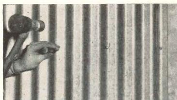
**4** Outer corrugated sheet is impaled over stud rivet extensions and secured by riveting over burrs placed on stud extensions.
