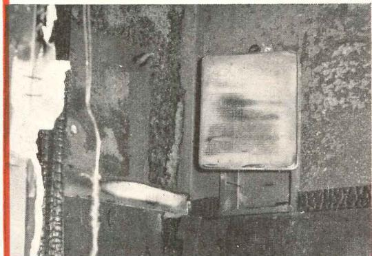
Nowhere has fire broken through the wall, although the tile panels are blistered.
