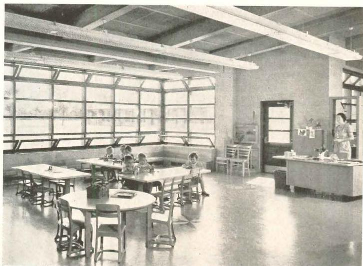
Classroom corridors in all three wings are double loaded, lined with lockers; roof is depressed to permit glass block clerestories giving bilateral lighting to all classrooms. Despite unusually heavy snow last year, roof troughs and skylights caused no trouble.
