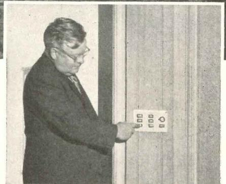
▲ A flush mounted switch in the living room controls all garden, yard and driveway lights. Wiring costs are held down in the G-E remote-control system because small, lightweight control wire is used to connect switches to relays. You can have as many switches as convenience dictates without increasing the cost prohibitively.
