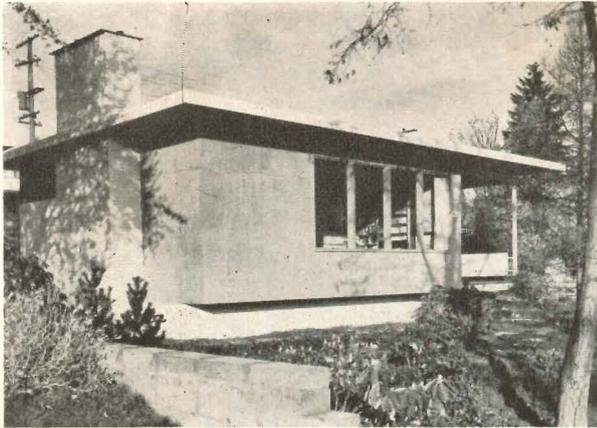
Exposed plywood exteriors find their way into commercial buildings as well as houses, witness these photos: (1) A combination of flat and curved plywood surfaces form the exterior skin for this small office building by Richard Neutra. (2) Small house by Paul Thiry with flush plywood covering. (3) Long length, scarf-jointed panels were set into the exterior framing members for this Information Center in Portland, Ore., which was designed by John Yeon
