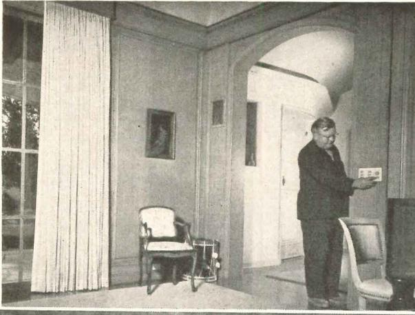
◀ Homeowner Sheriffs demonstrates the master selector switch in the living room that opens and closes draperies at the window. Switches also operate draperies in four other parts of the house. This master switch controls 8 additional circuits. There are five master selector switches in the Sheriffs home.
