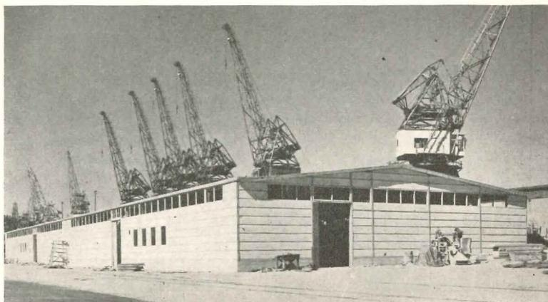
*Above, right: this warehouse building was constructed with roof slabs of the material. Below, left and right: construction shots illustrate ease of installation, made possible by the light weight of the slabs*
