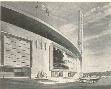
Above, left and right: section and plan of the pool building. Left: sketch of winning design in stadium competition. Designed for construction with both prestressed and steel-reinforced concrete, it accommodates 125,000 people
