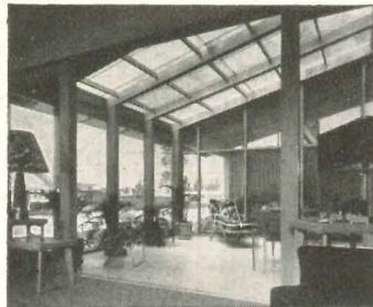
Resolite is a rugged structural sheet of Fiberglas-reinforced resin plastic, flat or corrugated for added structural strength. The material is unaffected by weather extremes of heat, cold or moisture. It will not rust, oxidize, mildew or rot. It is simple to apply with screws or nails and with ordinary tools and skill; it is easily adapted to roof, wall or partition.
