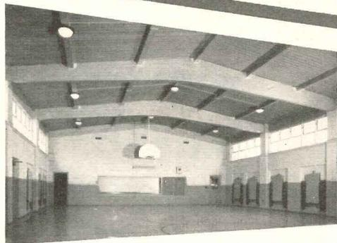
The natural beauty of Rilco glued laminated wood gives an attractive interior; the ease of erection and elimination of interior finishing cuts construction costs—yet Rilco structural members offer the architect freedom of design with simple yet effective construction in a fire-resistant material.
