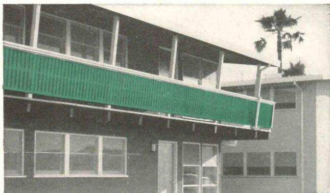
CHEM-O-GLAS (pronounced Kem-O-Glass) is precision molded in 8' lengths, 32 1/2" wide, (32" wide from c/c of outside ribs when overlapped.) Some jobber-dealer territories still open.
